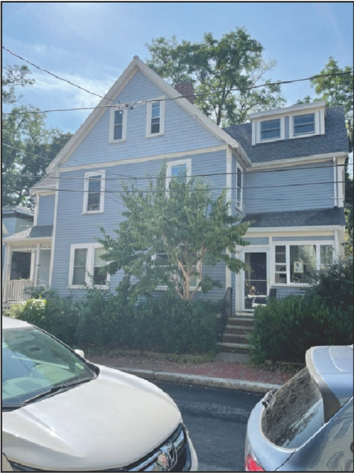
Front View from Northwest Corner
