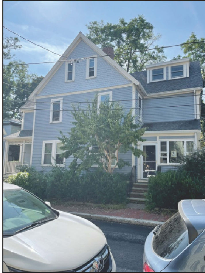
Front View from Northwest Corner
