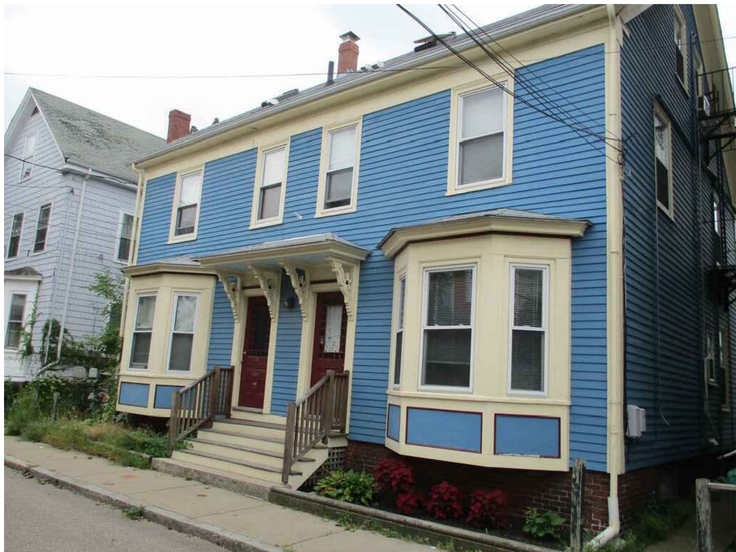
0-2 FAIRMONT AVE STREET VIEW - NO CHANGE
