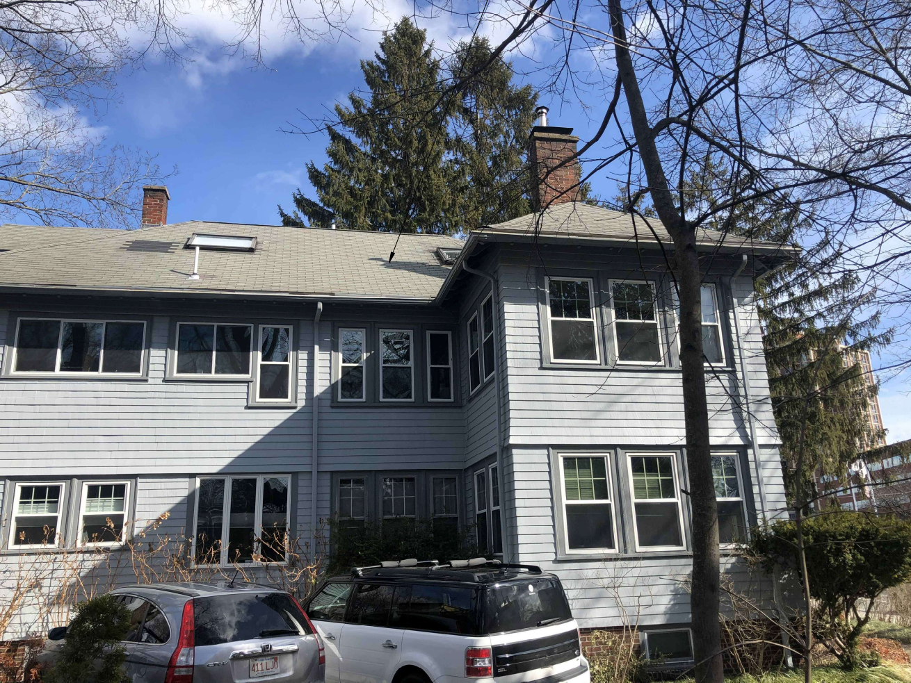
321 Mt Auburn St - VIEW FROM LEFT SIDE YARD
