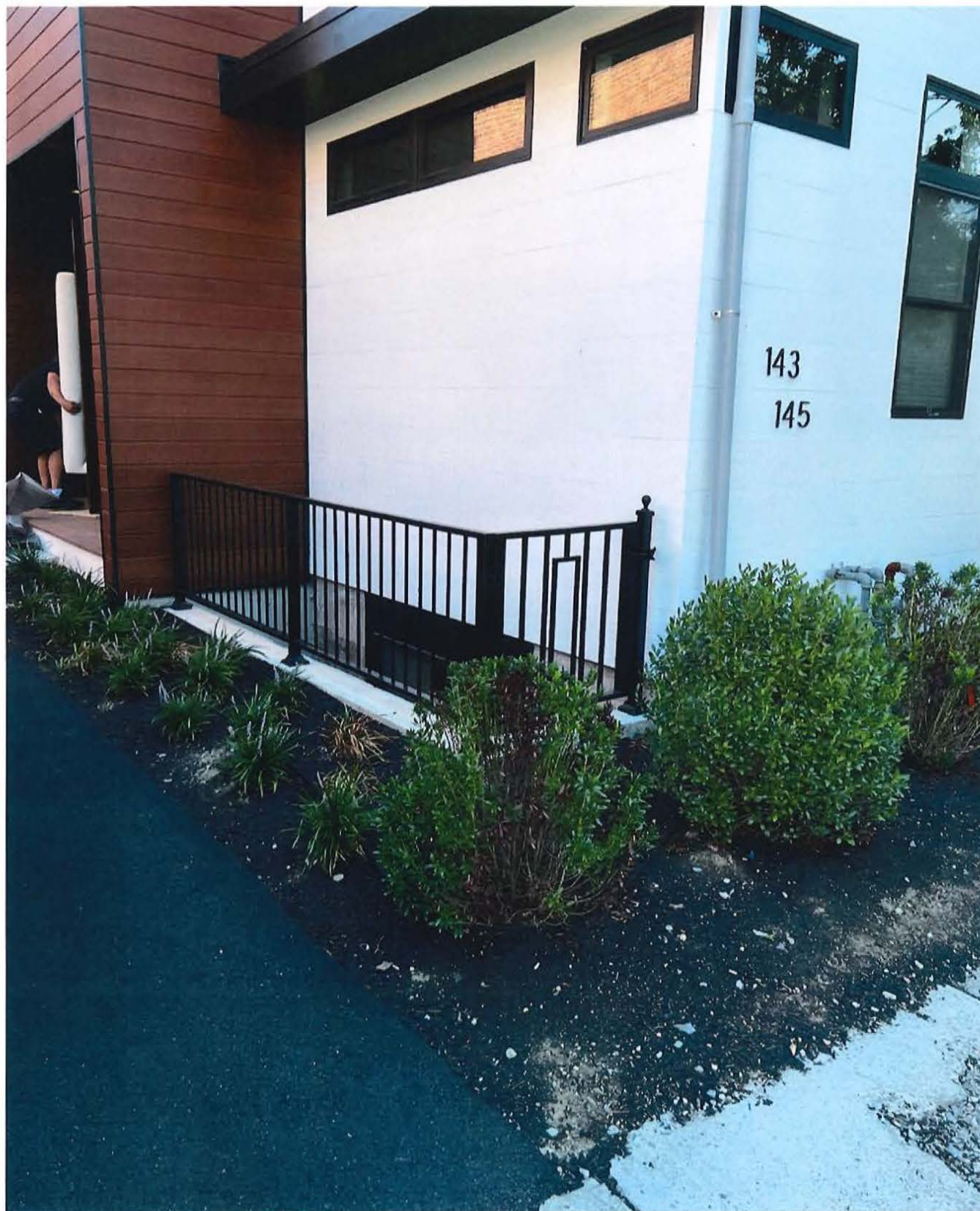
Window well with railing located only a few feet (~3 ft) from the sidewalk.
