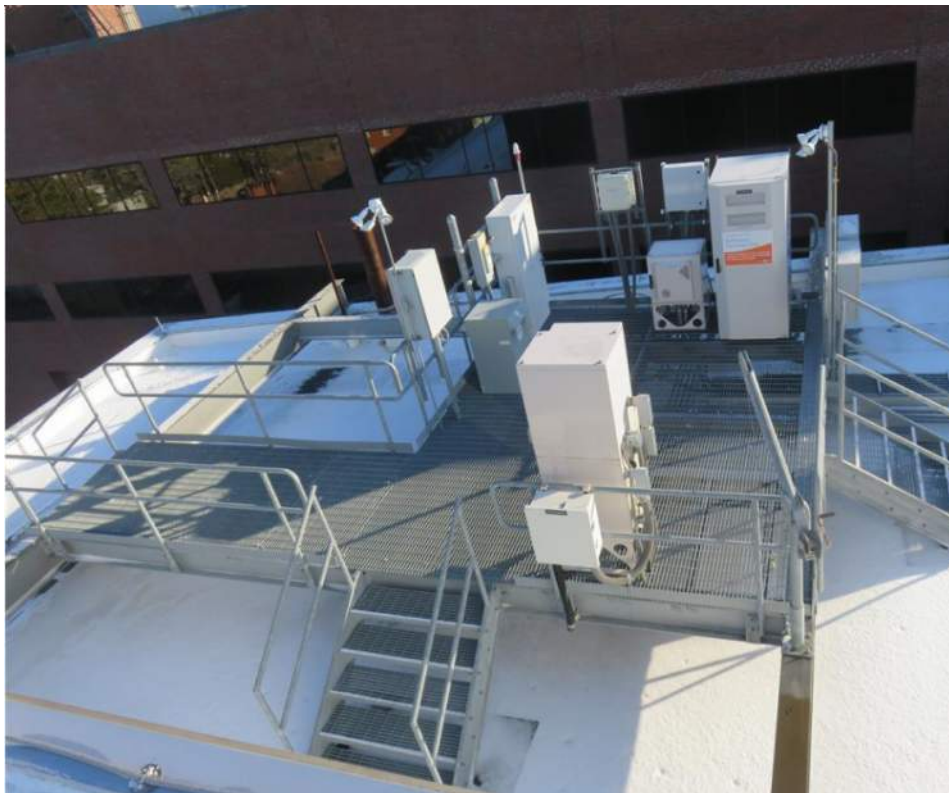
Photo 6: Sample photo illustrating the existing equipment platform.
