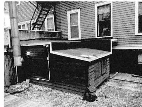
EXISTING ATTACHED UTILITY STRUCTURE
