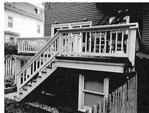
EXISTING DECK NEXT DOOR
