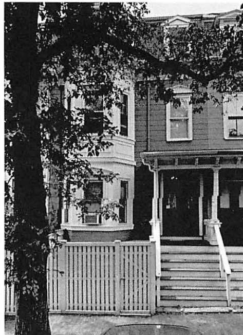
FRONT OF BUILDING
