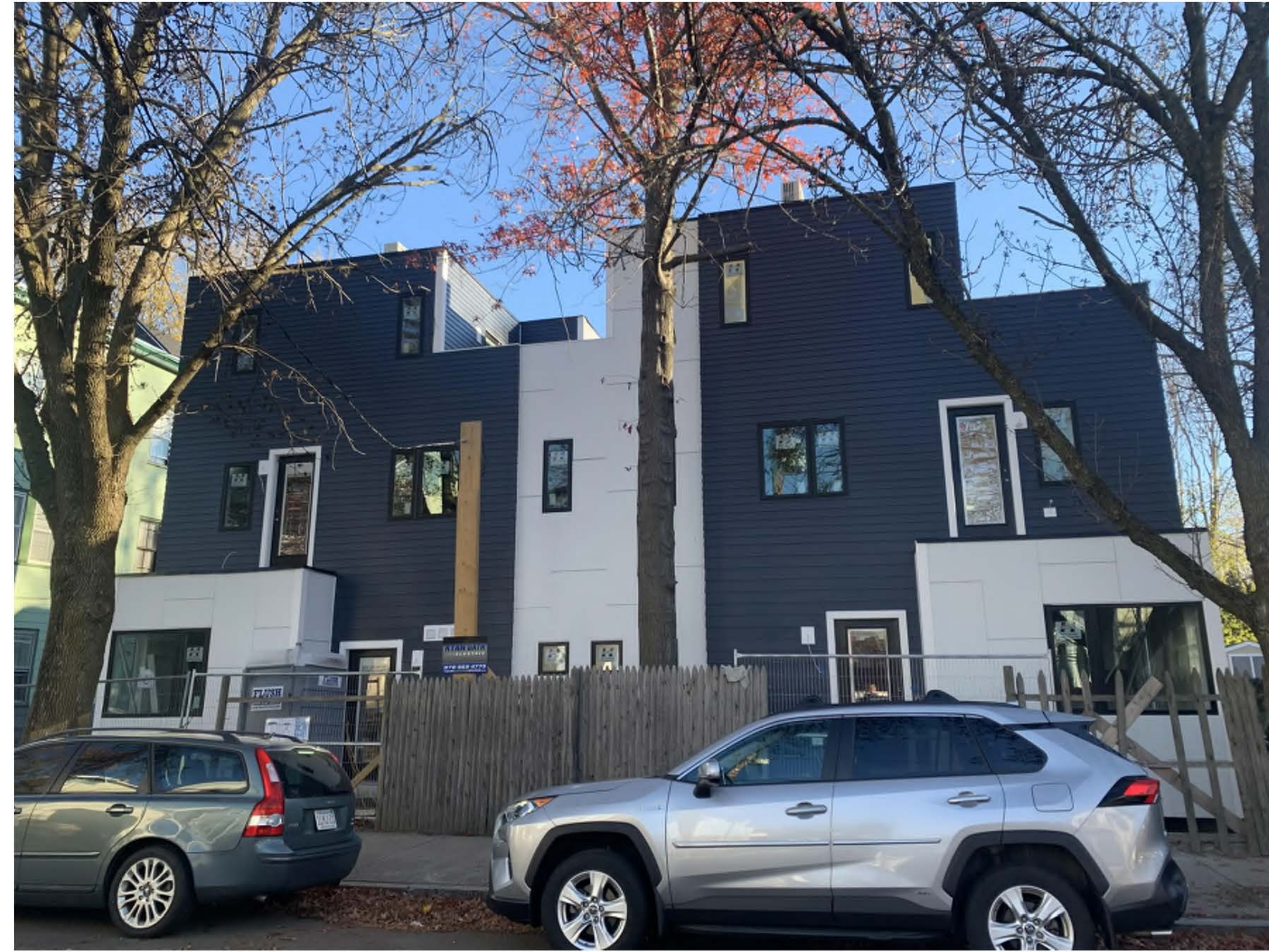
41 WEBSTER - EXISTING CONDITION
