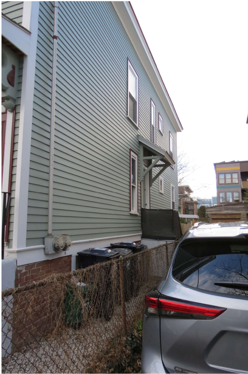
35 Kinnaird - north side from front
