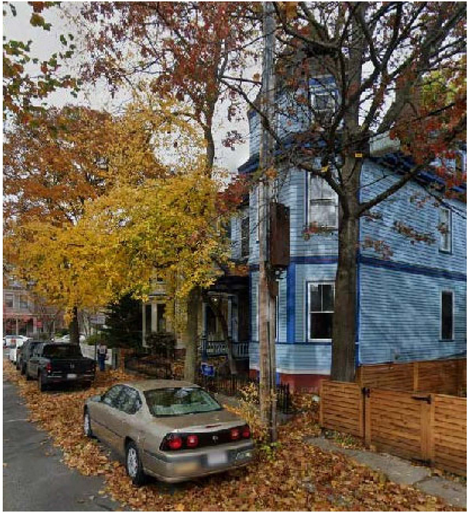
EXISTING PHOTO FRONT SW CORNER
