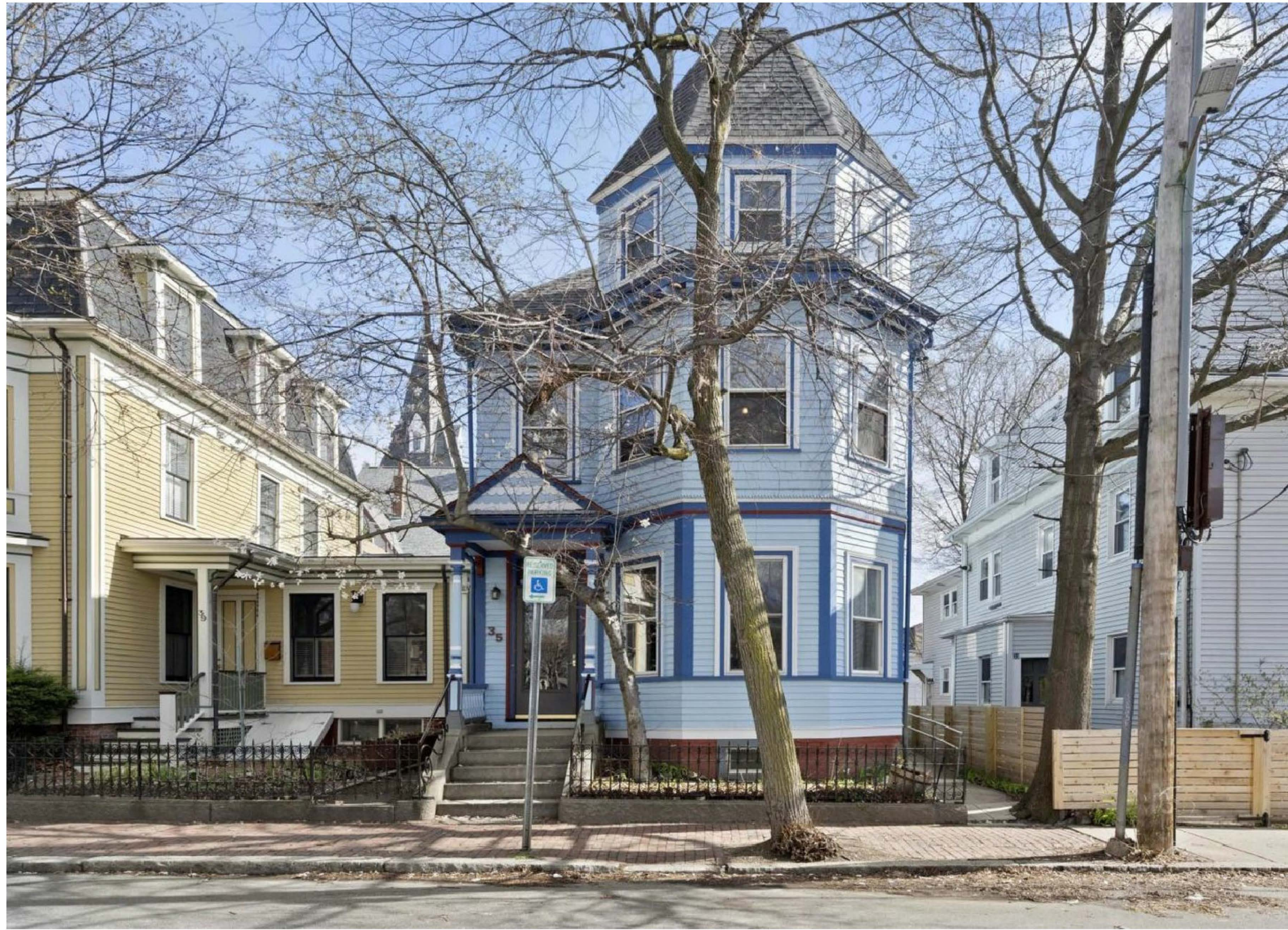
EXISTING PHOTO AT LAWRENCE STREET
