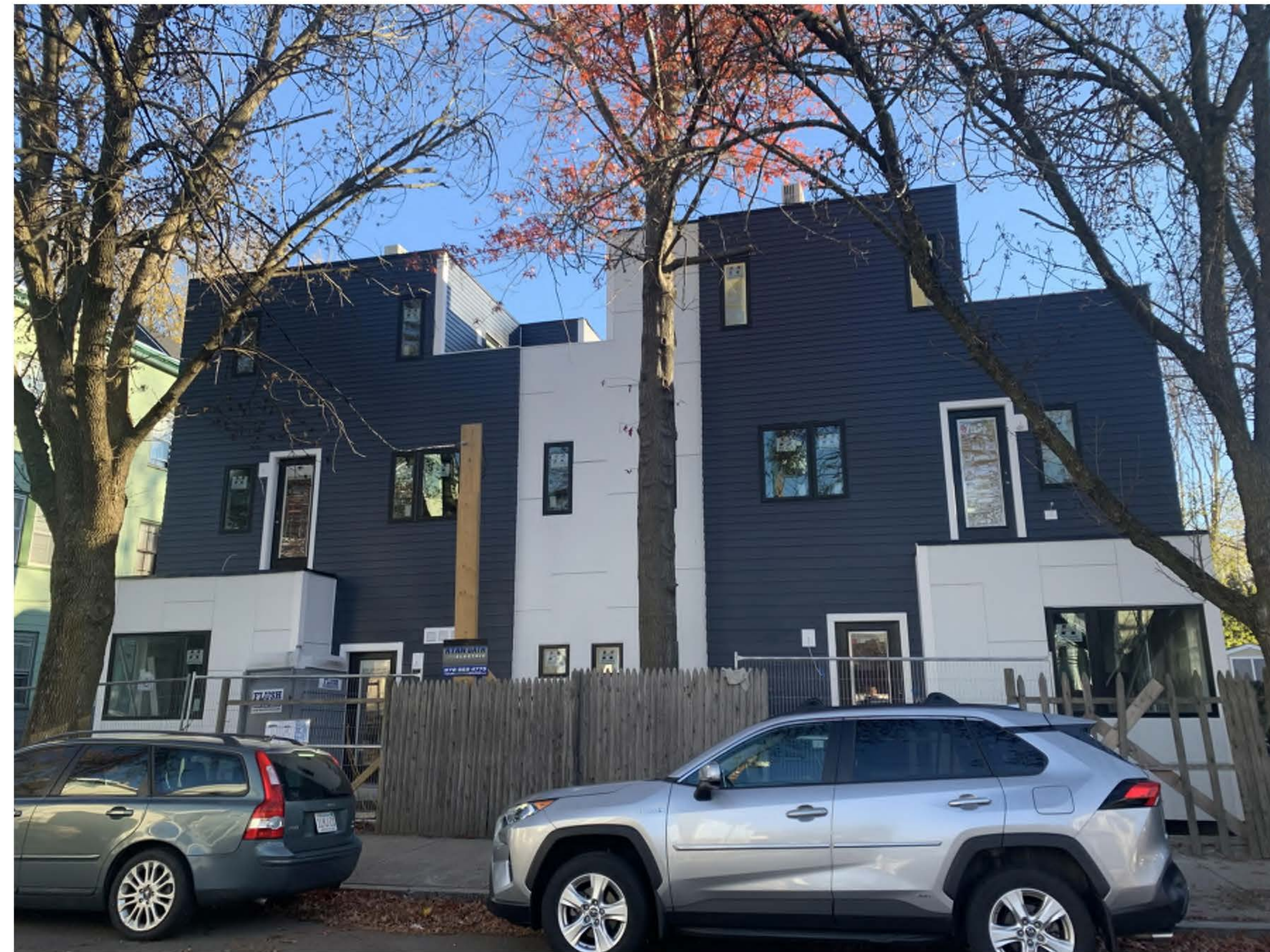
41 WEBSTER - EXISTING CONDITION
