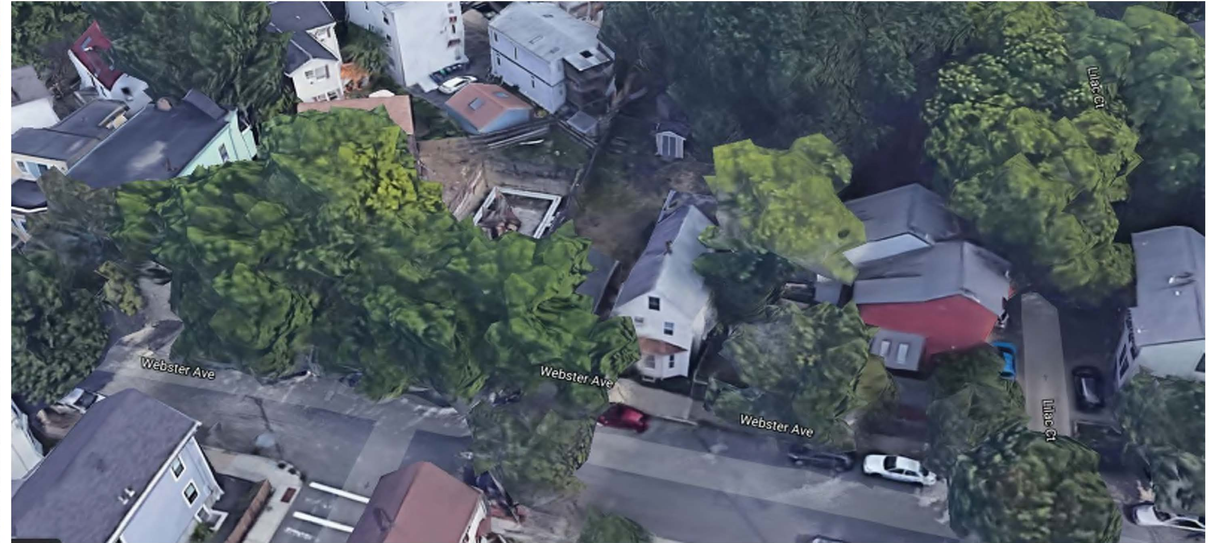
33 - 35 WEBSTER PERSPECTIVE VIEW - EXISTING CONDITION
