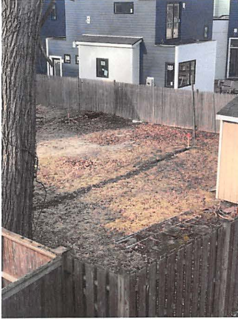
Figure 1: Root pruning undertaken in December 2021, visible as unvegetated line in the backyard of 33-35 Webster ave. Picture taken Jan 22, 2022
