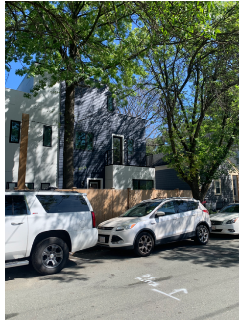
33-35 Webster Ave streetscape AFTER 2021-22 nearby home construction
