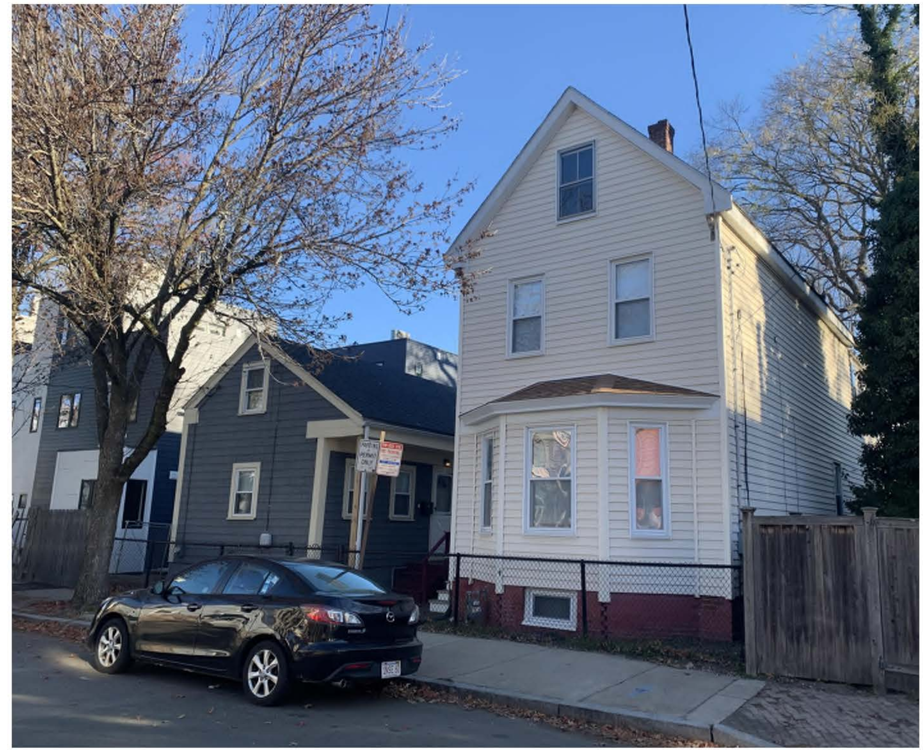
33 - 35 WEBSTER - EXISTING CONDITION
