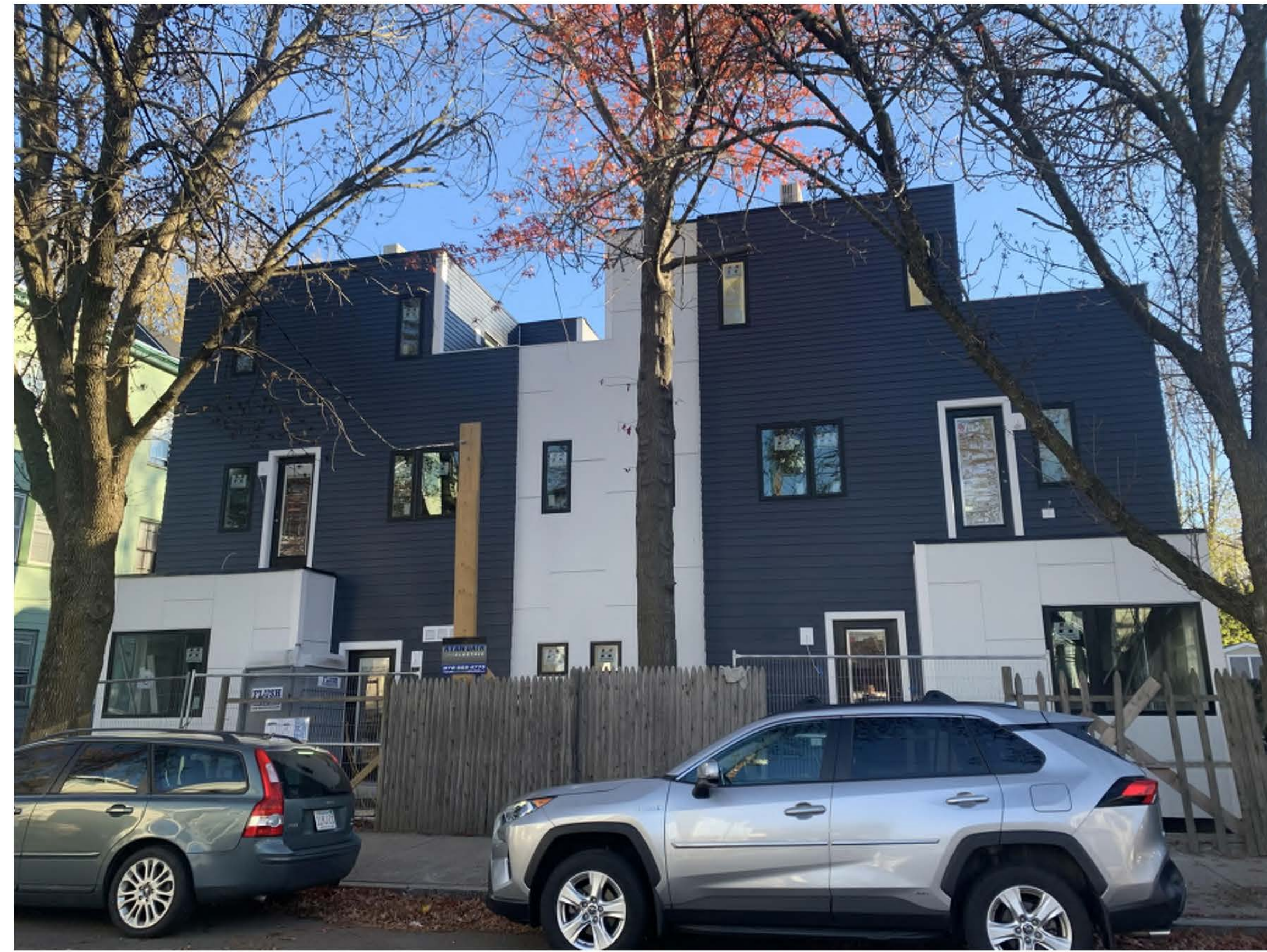
41 WEBSTER - EXISTING CONDITION
