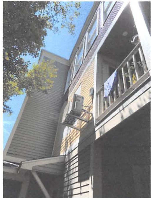
Rear Elevation Showing all 3 Porches 1st floor enclosed, expanded into rear 2nd floor partially enclosed 3rd totally enclosed and full height windows
