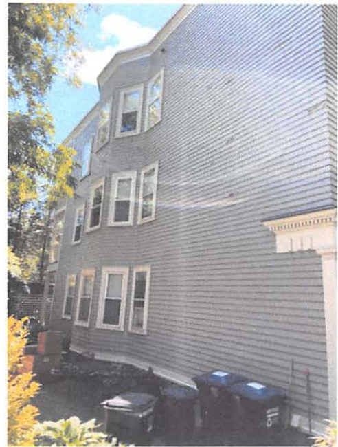
Left Elevation Also rear yard
