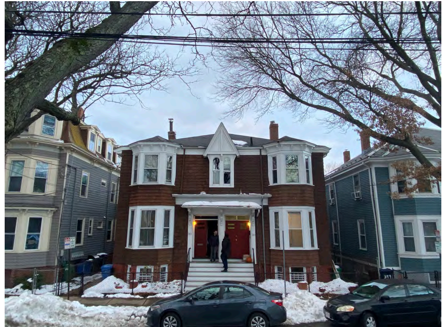
EXISTING STREET VIEW
