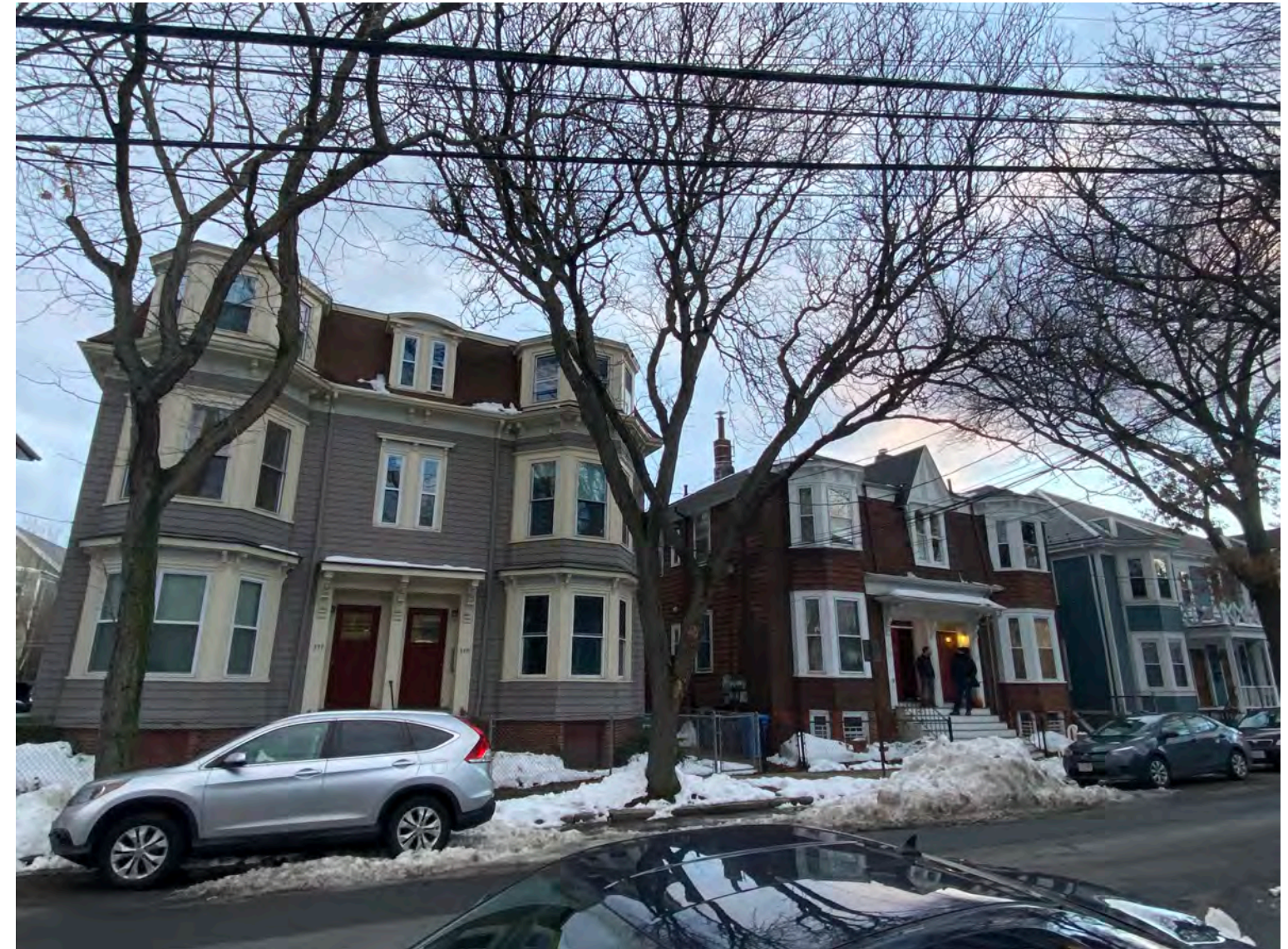
EXISTING STREET VIEW
