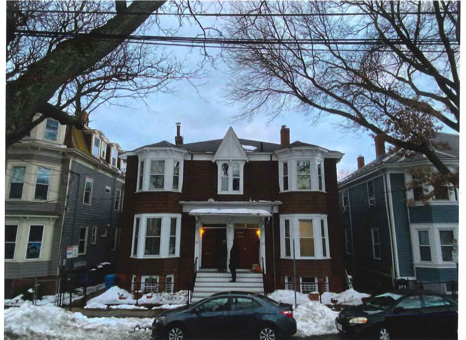
EXISTING STREET VIEW
