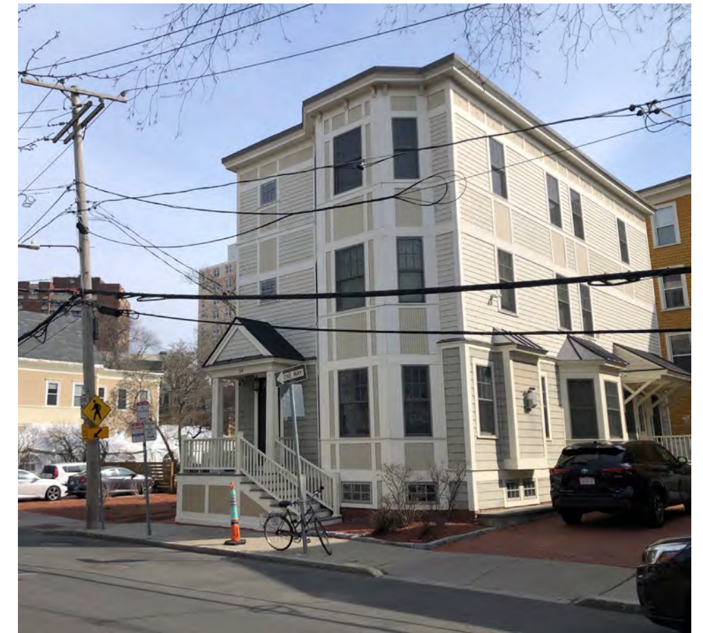
Current Condition: South / West Elevation
