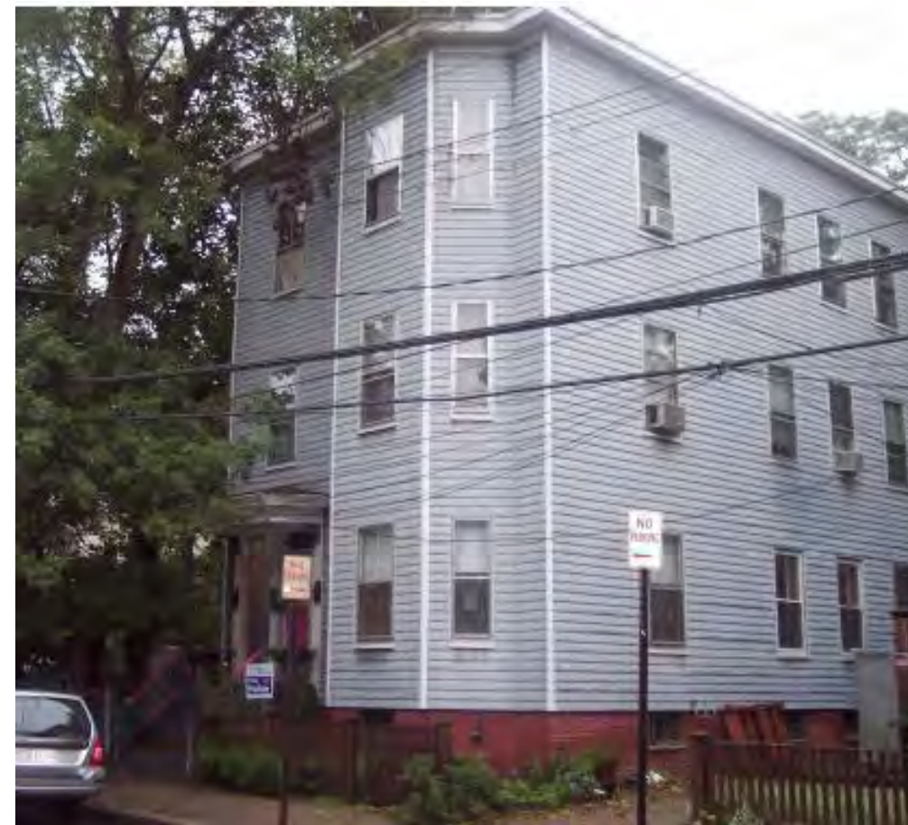
Pre-Renovation Condition: West Elevation
