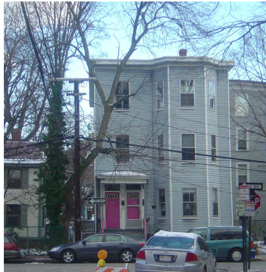
Pre-Renovation Condition: West Elevation
