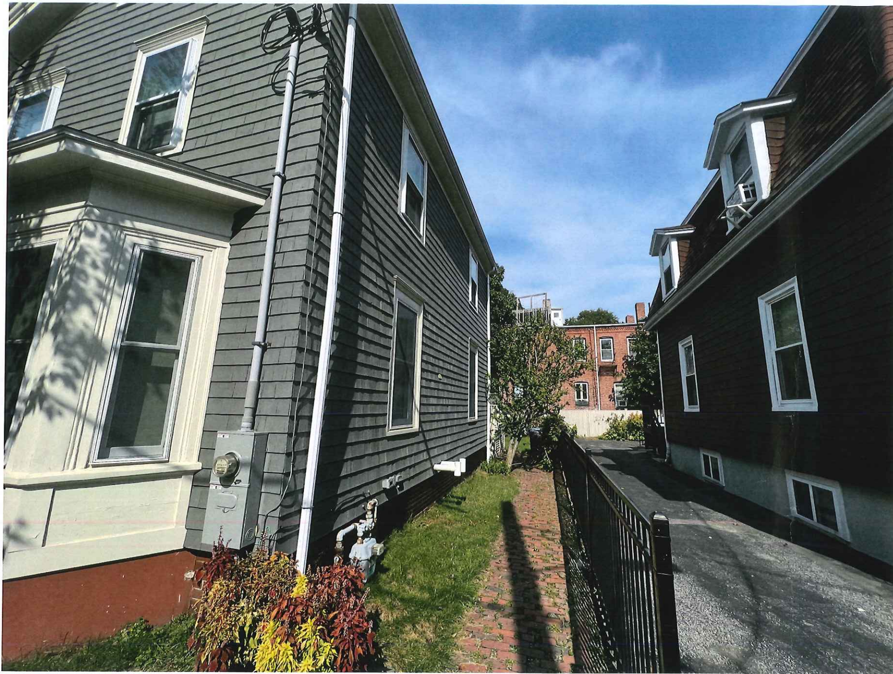
3 AMORY PLACE VIEW OF RIGHT SIDE YARD FROM FRONT,
