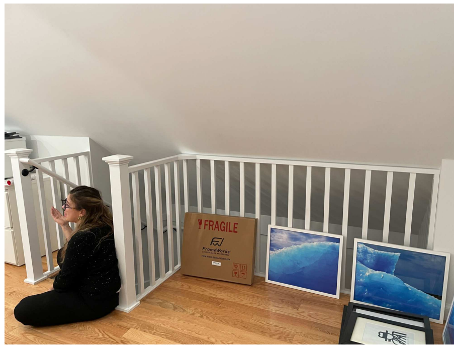
EXISTING ACCESS TO THE ATTIC
