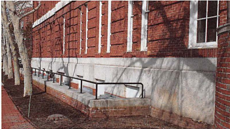
Areaway at James Street
