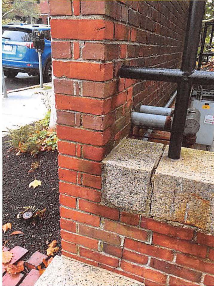
Existing Extended Wall at North End
