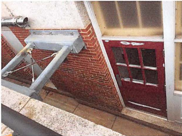
Areaway Entry to Schlesinger Basement and Structural Bracing
