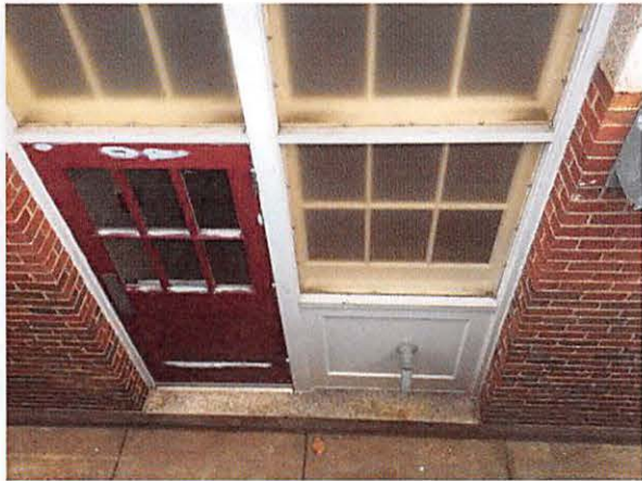
Areaway Entry to Schlesinger Basement
