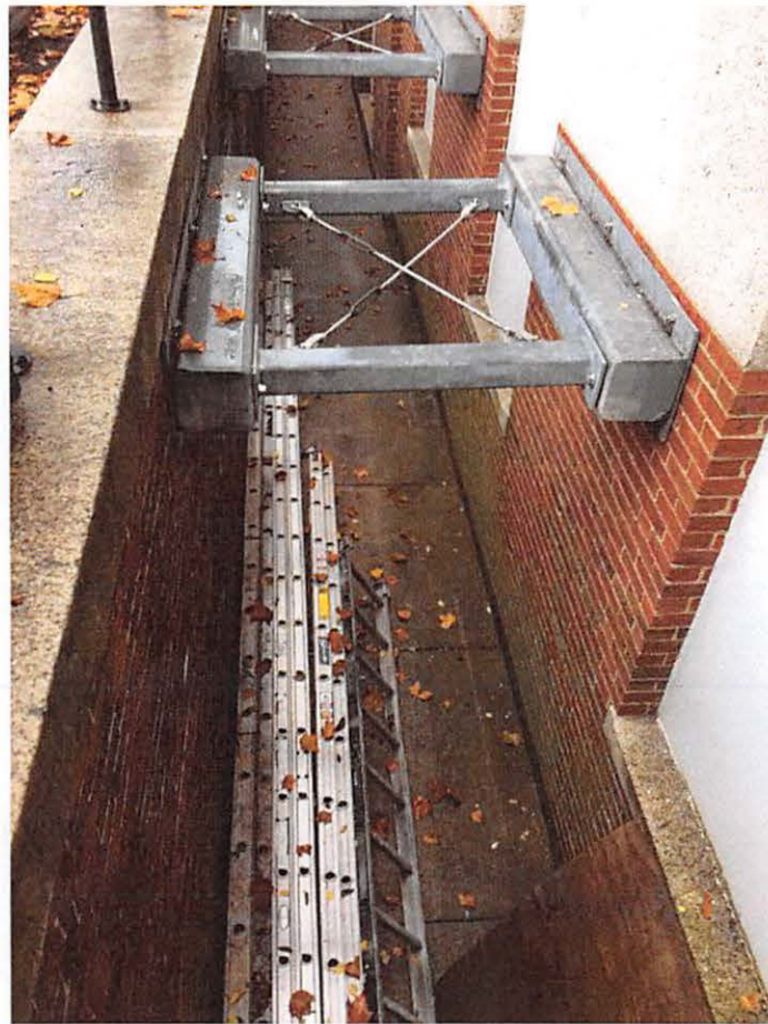
View into Areaway at Proposed Location for Material Lift
