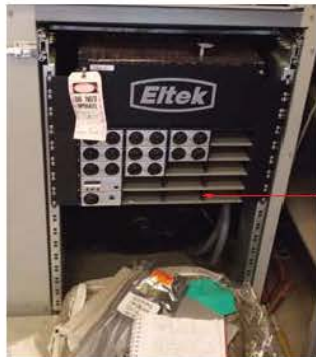
FRONT VIEW EXISTING RECTIFIER RACK SCALE: NTS
