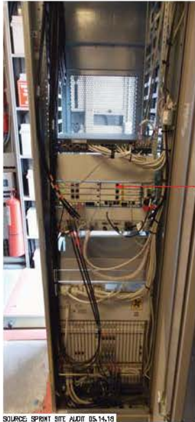
FRONT VIEW EXISTING MM-BTS EQUIPMENT CABINET SCALE: NTS
