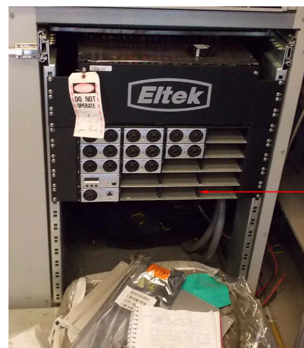
FRONT VIEW EXISTING RECTIFIER RACK 3 SCALE: NTS
