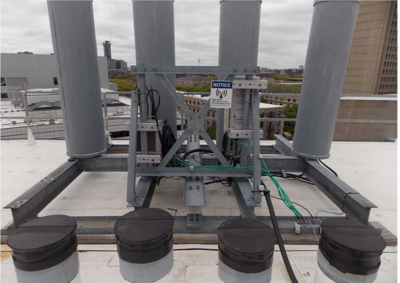
Existing Beta Sector Antenna Frame
