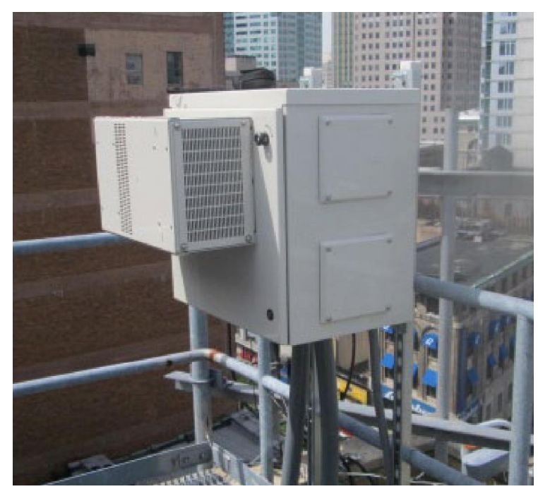
EMERSON NETXTEND COMPACT 2416 FIBER CABINET DIMENSIONS: 24.0"H x 24.0"W x 25.2"D WEIGHT: 64 lbs QUANTITY: TOTAL OF 1
