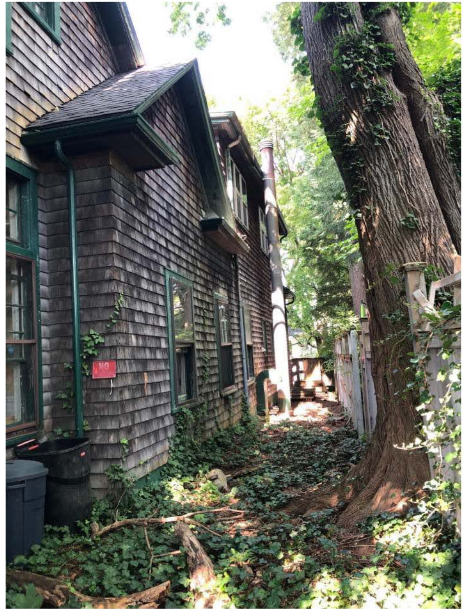
40 RESERVOIR ST. EXISTING CONDITIONS
