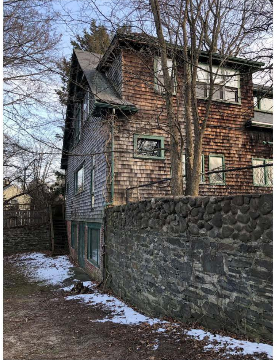
40 RESERVOIR ST. EXISTING CONDITIONS
