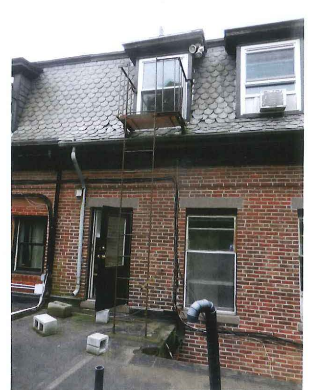
REAR FACADE- 2ND FLOOR
