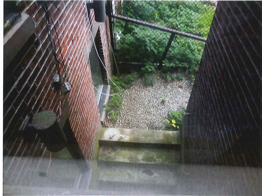
BASEMENT ENTRANCE AT THE REAR
