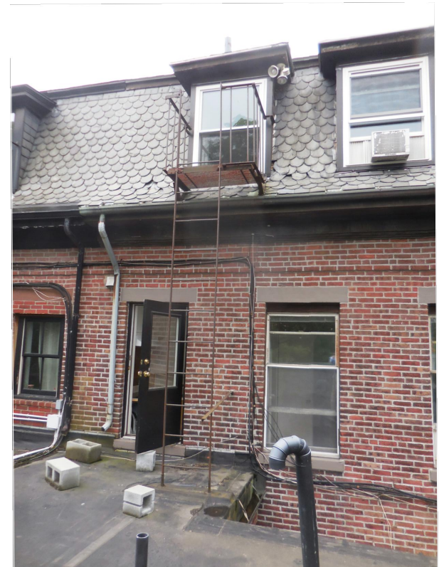
REAR FACADE- 2ND FLOOR
