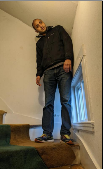
3RD FLOOR STAIR HEIGHT & CLEARANCE ISSUES
