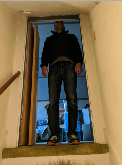
3RD FLOOR STAIR HEIGHT & CLEARANCE ISSUES
