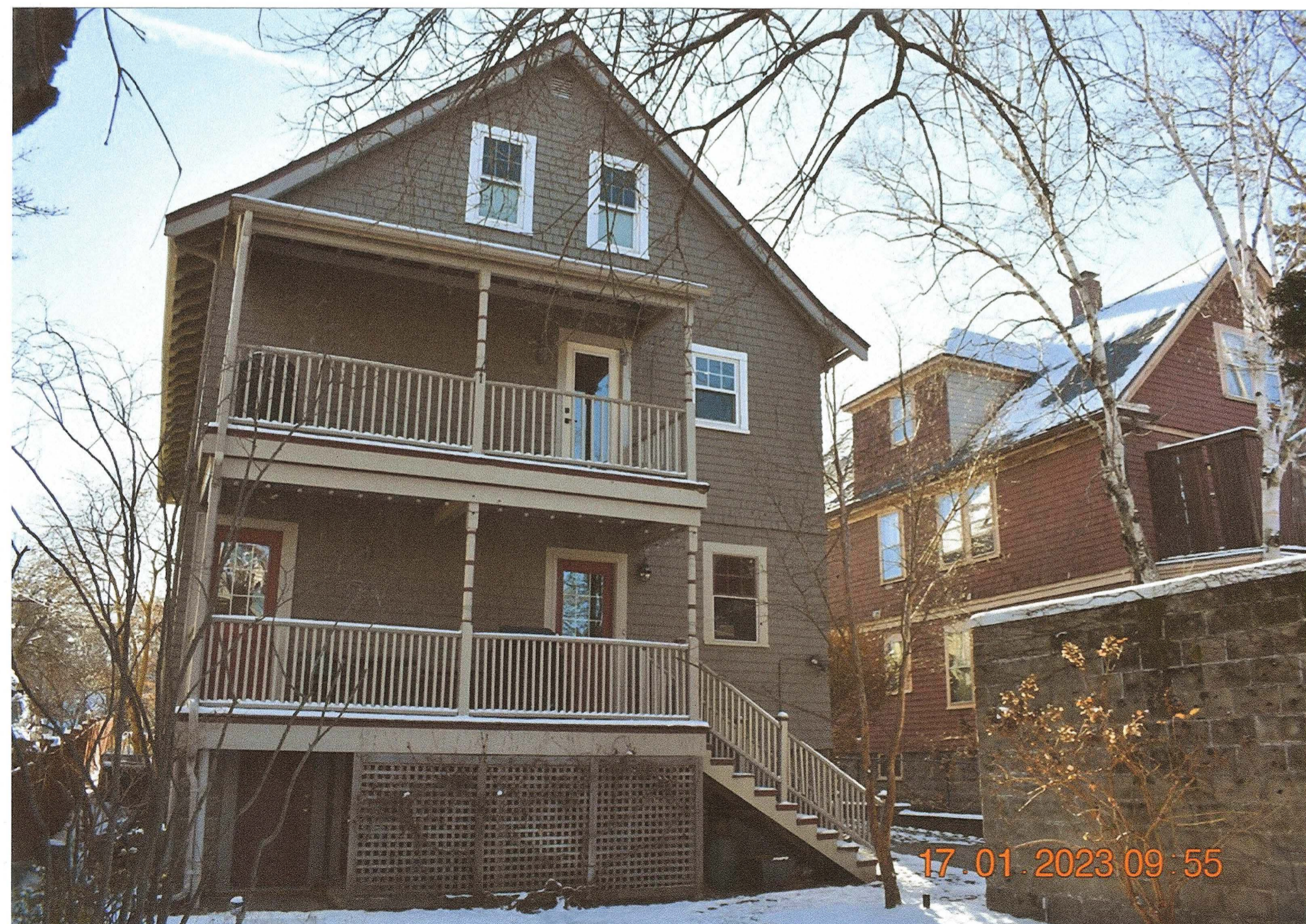
EXISTING REAR PORCH
