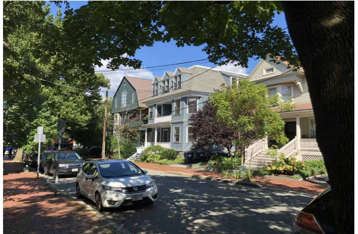
STREET VIEW FROM RIGHT SIDE
