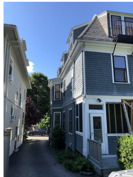
DRIVEWAY SIDE ELEVATION FROM REAR YARD
