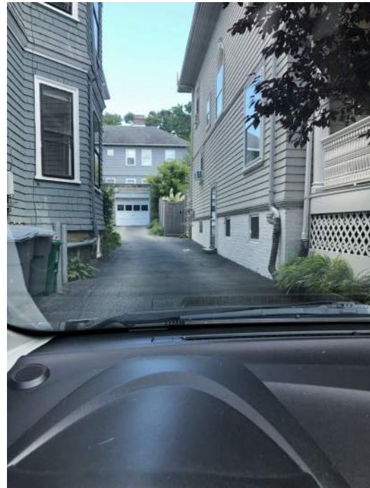
VIEW OF ACCESSORY GARAGE STRUCTURE
