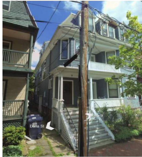
STREET VIEW FROM LEFT SIDE
