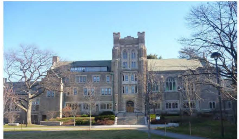
West Elevation from courtyard
