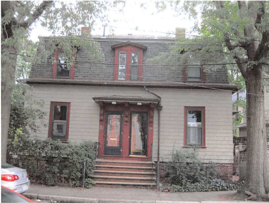
West Elevation from Kinnaird Street
