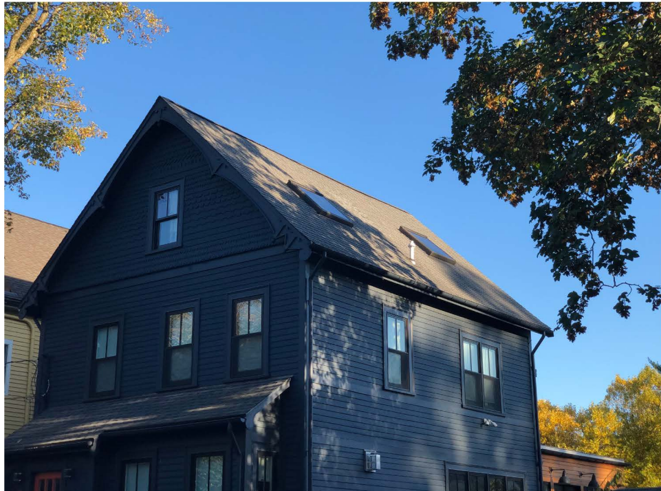
VIEW OF SKYLIGHTS TO BE REMOVED AND REPLACED BY DORMERS
