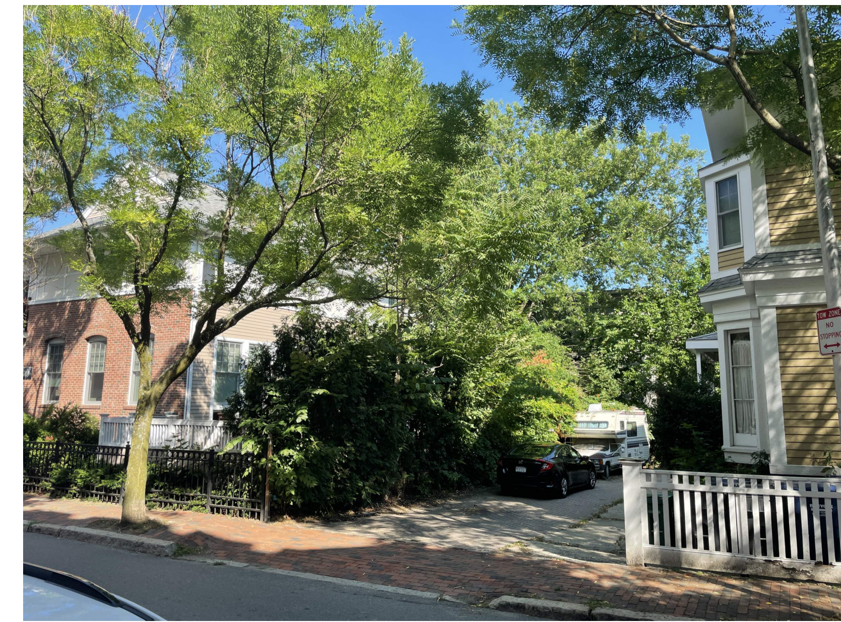
VIEW SHOWING VEGETATION SCREEN AND DRIVEWAY SEPARATING NEIGHBORING BUILDING
