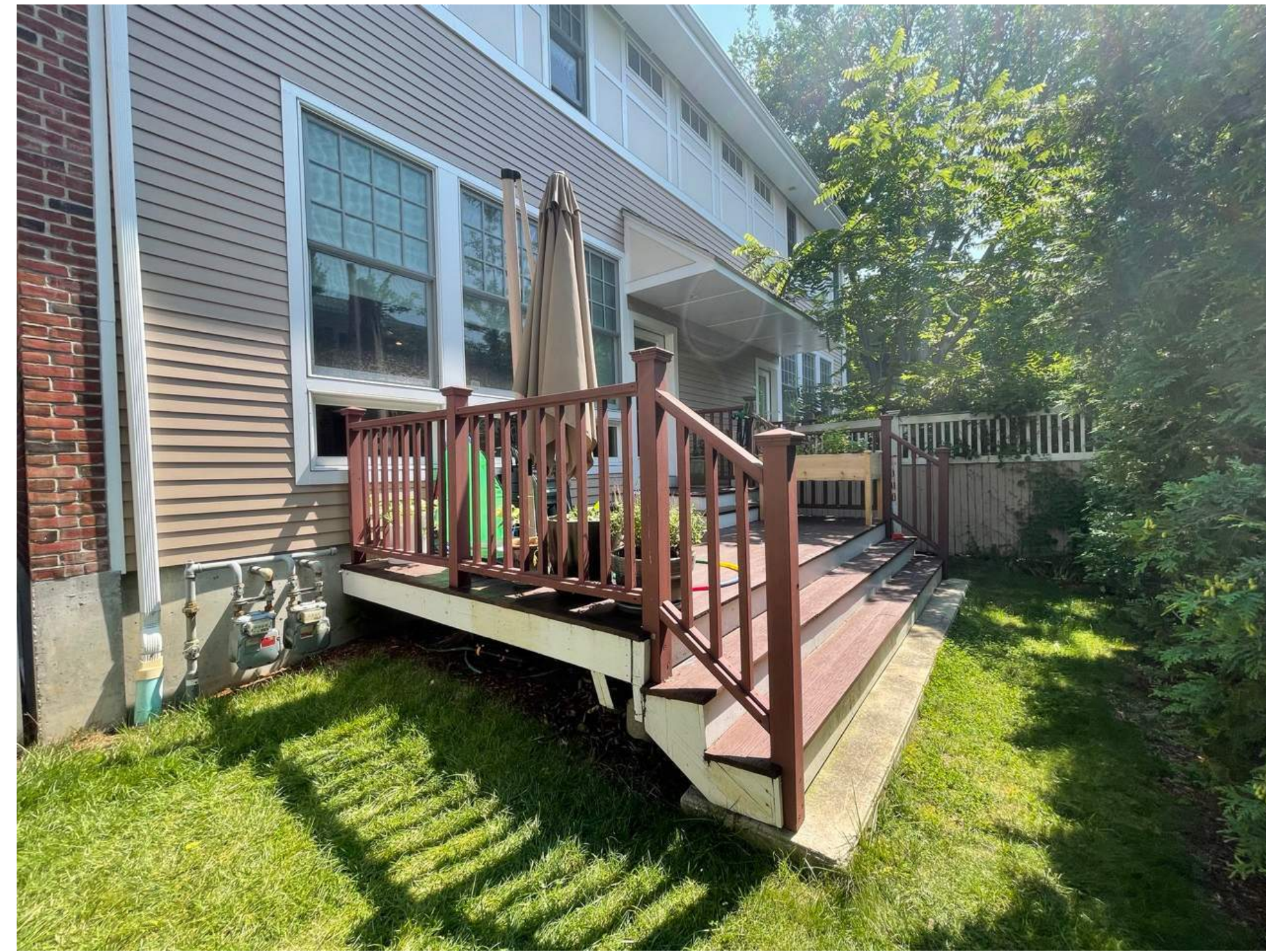
VIEW OF EXISTING DECK FROM YARD AREA
