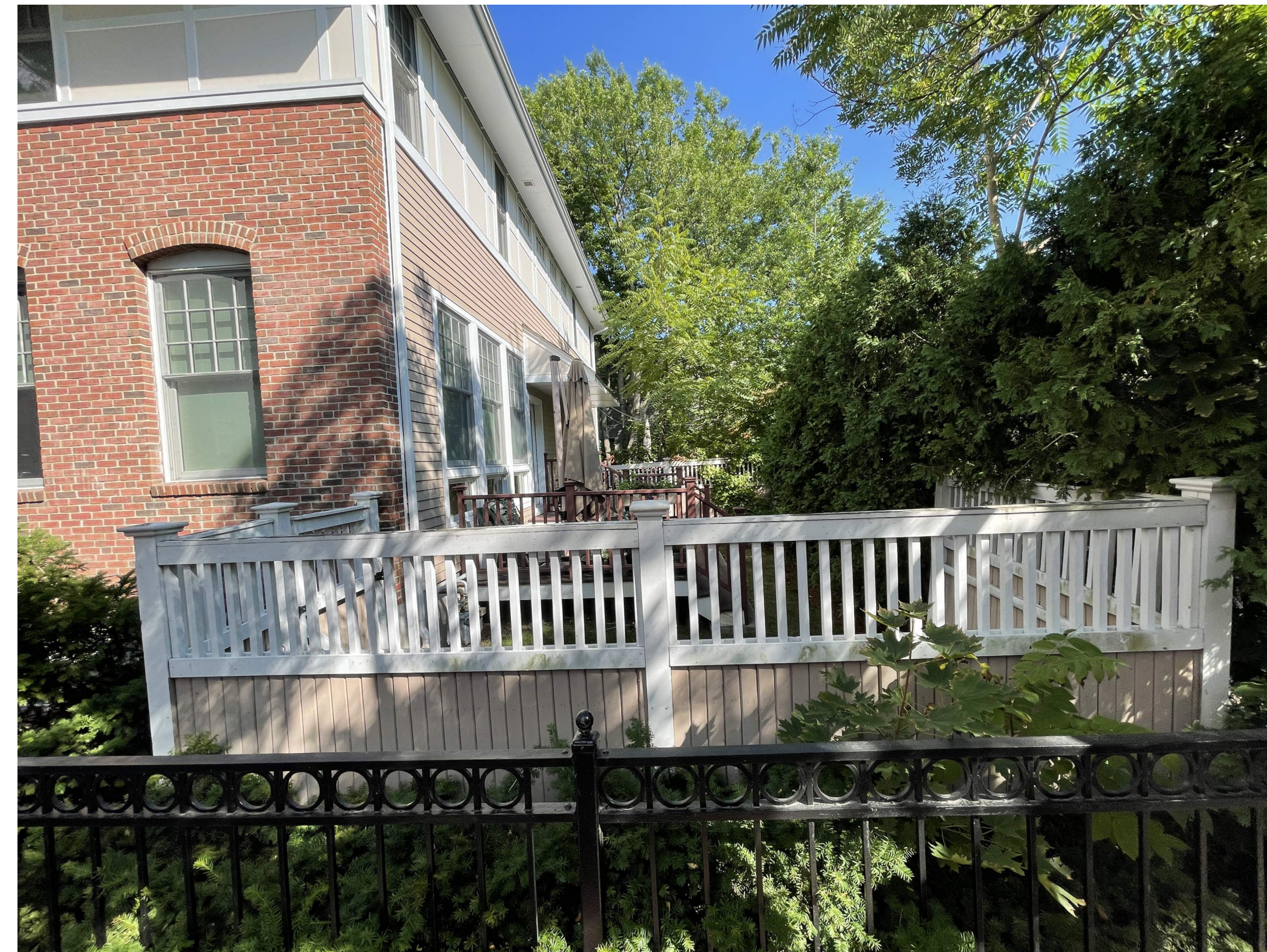
VIEW FROM STREET. UNIT 44 DECK IS IN THE REAR
