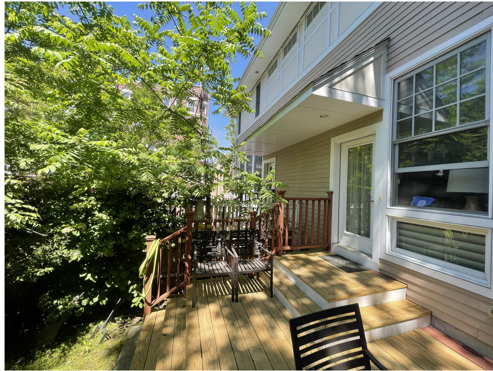
VIEW OF EXISTING DECK
