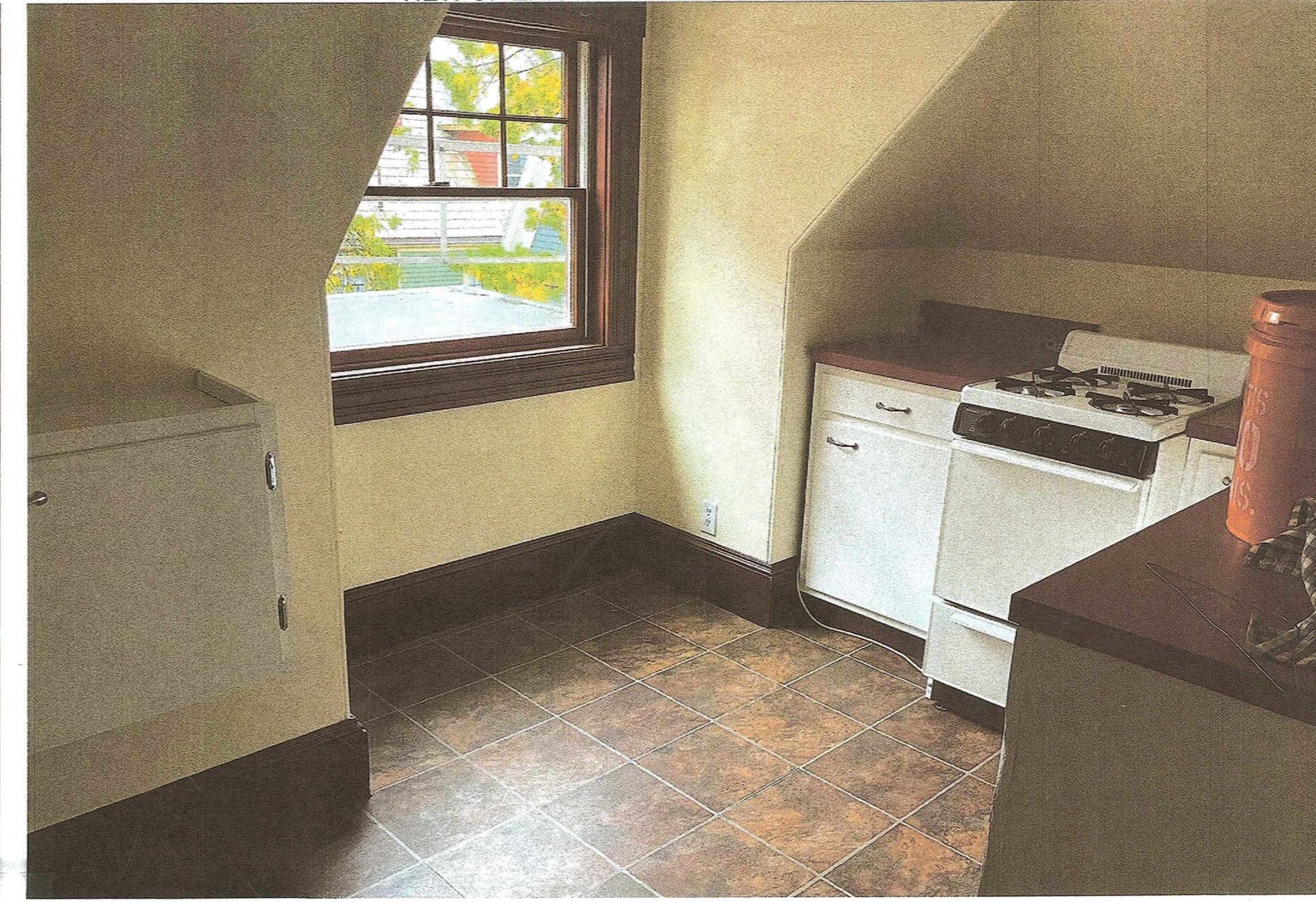
EXISTING 3 RD FLOOR APARTMENT KITCHEN
