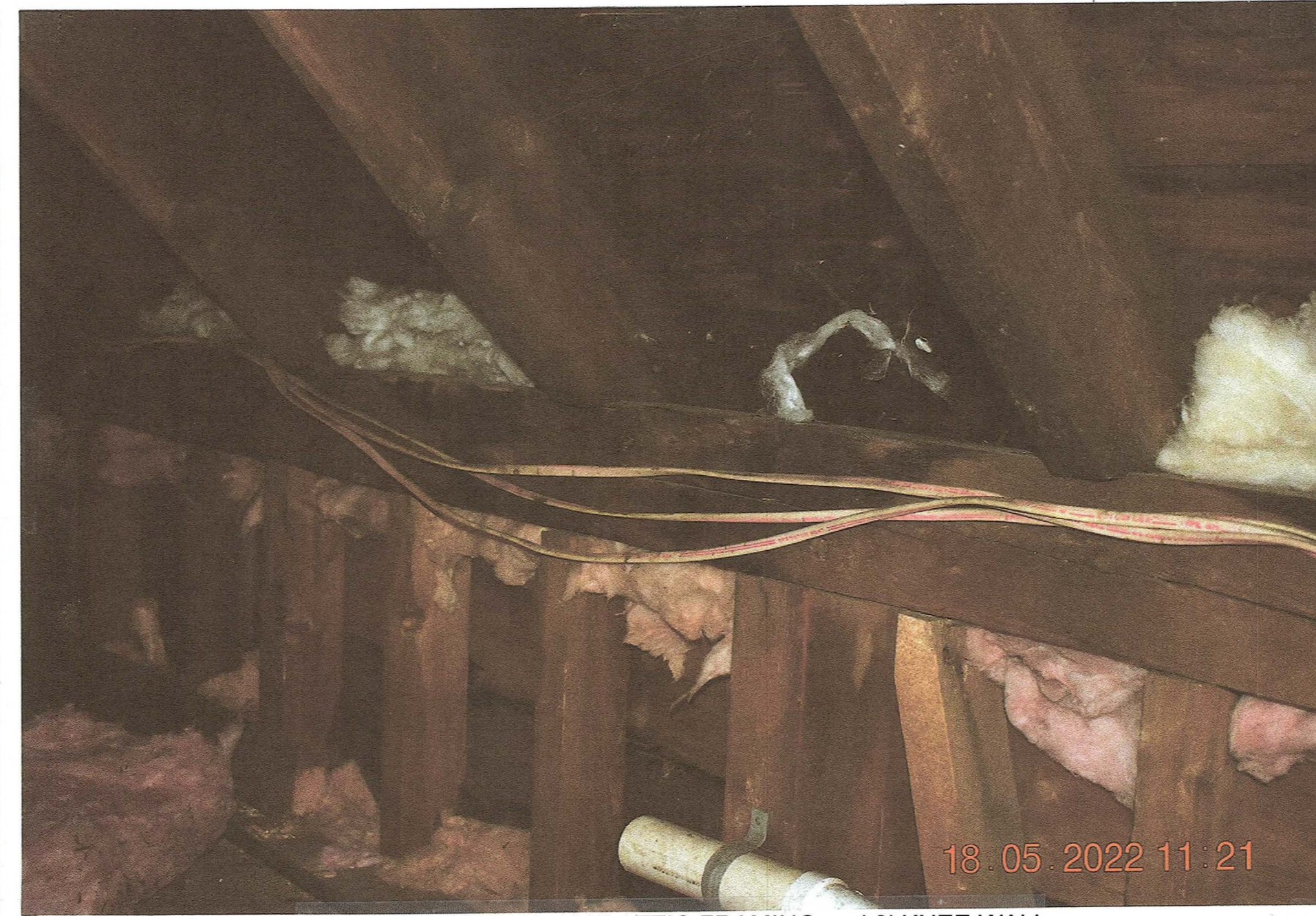
VIEW OF ORIGINAL 1895 ATTIC FRAMING and 2' KNEE WALL
