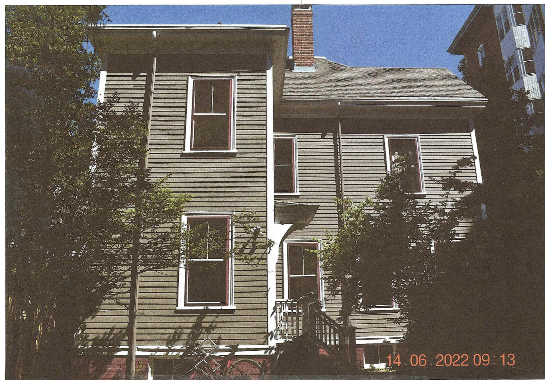
VIEW OF EXISTING SOUTH ELEVATION FROM REAR YARD
