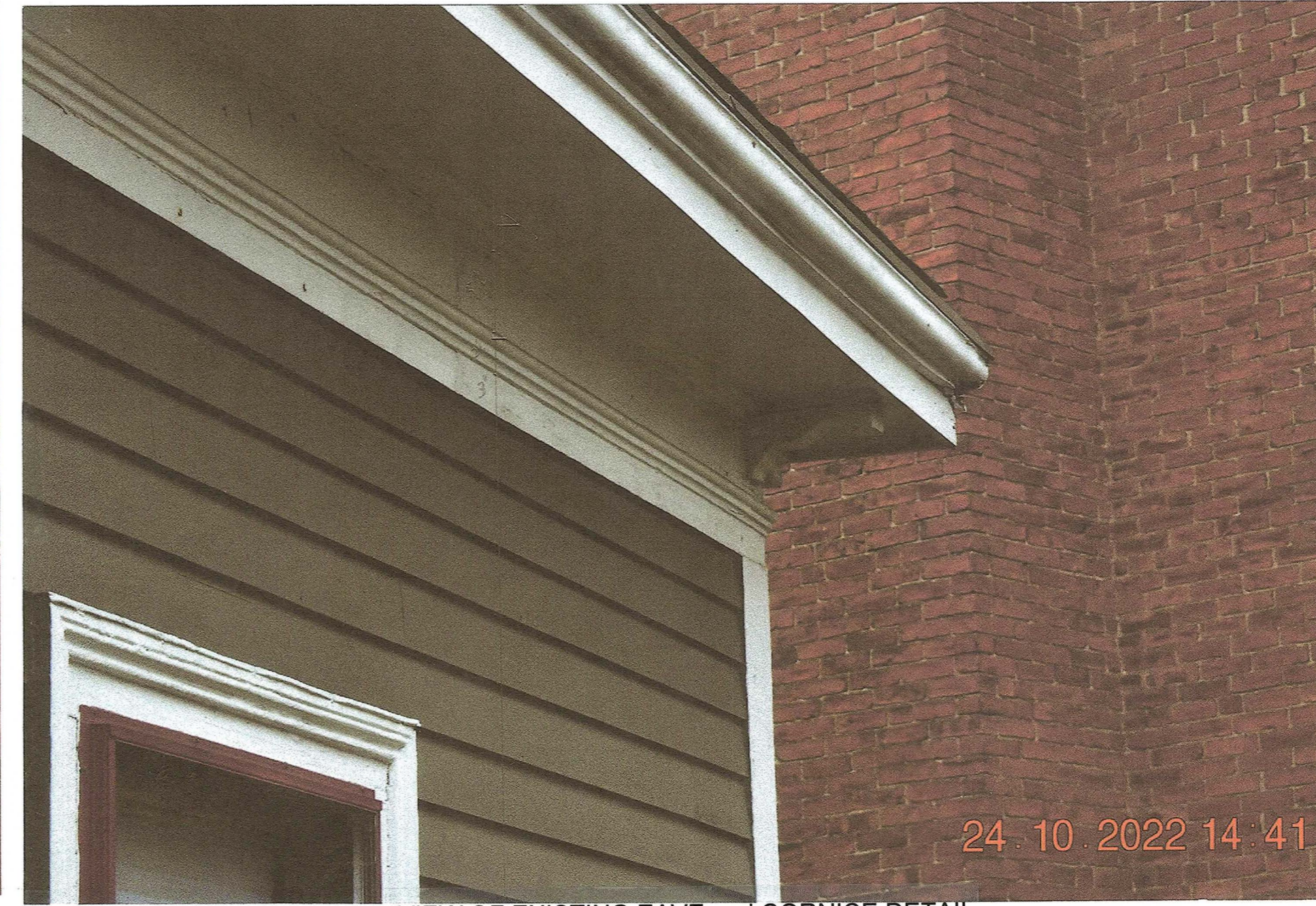
VIEW OF EXISTING EAVE and CORNICE DETAIL
