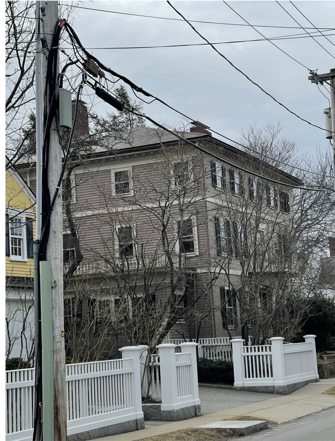
VIEW TOWARDS LEFT SIDE OF HOUSE
