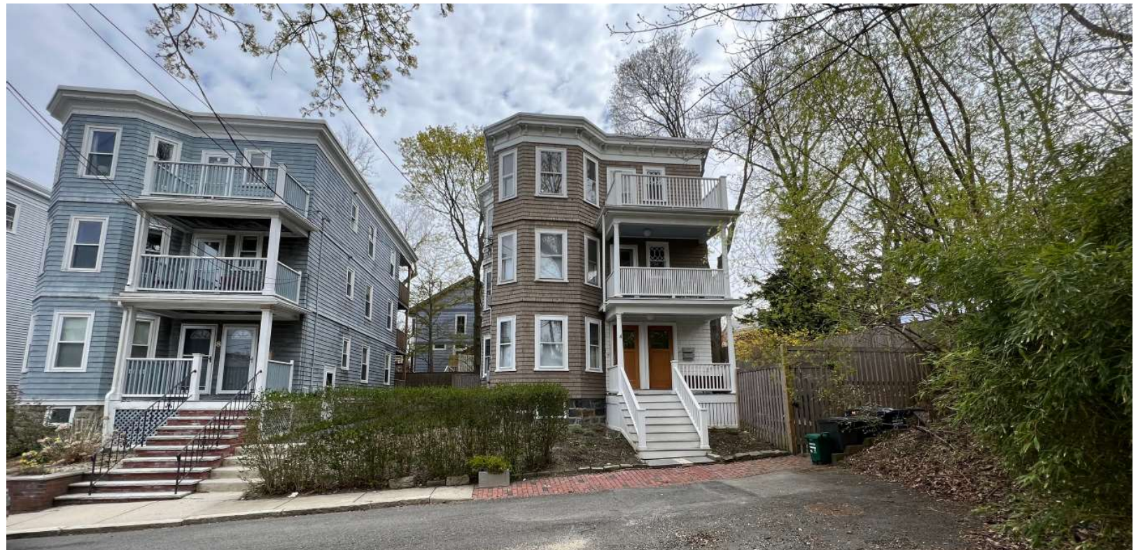
3) STREET SIDE VIEW OF 4 AND 6 WINSLOW PROPERTIES WITH EXISTING CURB CUT
