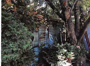
**Side View:** Facing 508 Franklin. Significant rust on roof and siding. Missing window.
