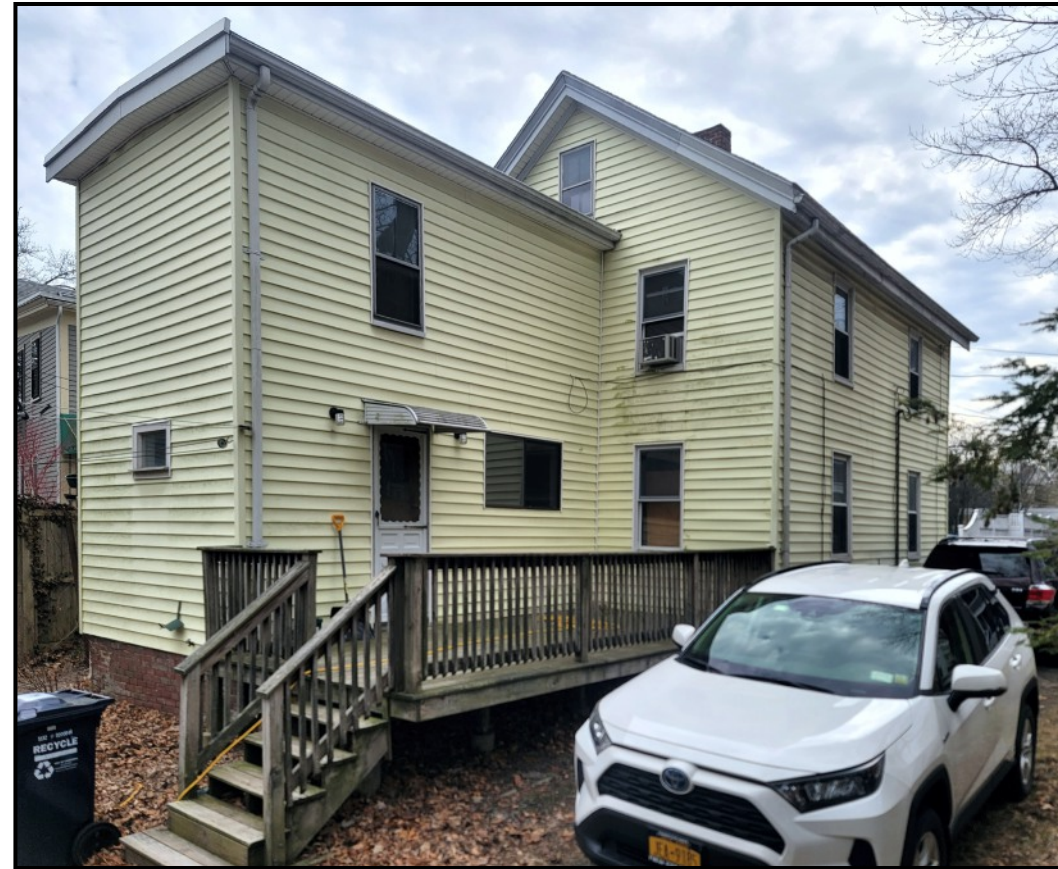
NE - Back Facade
