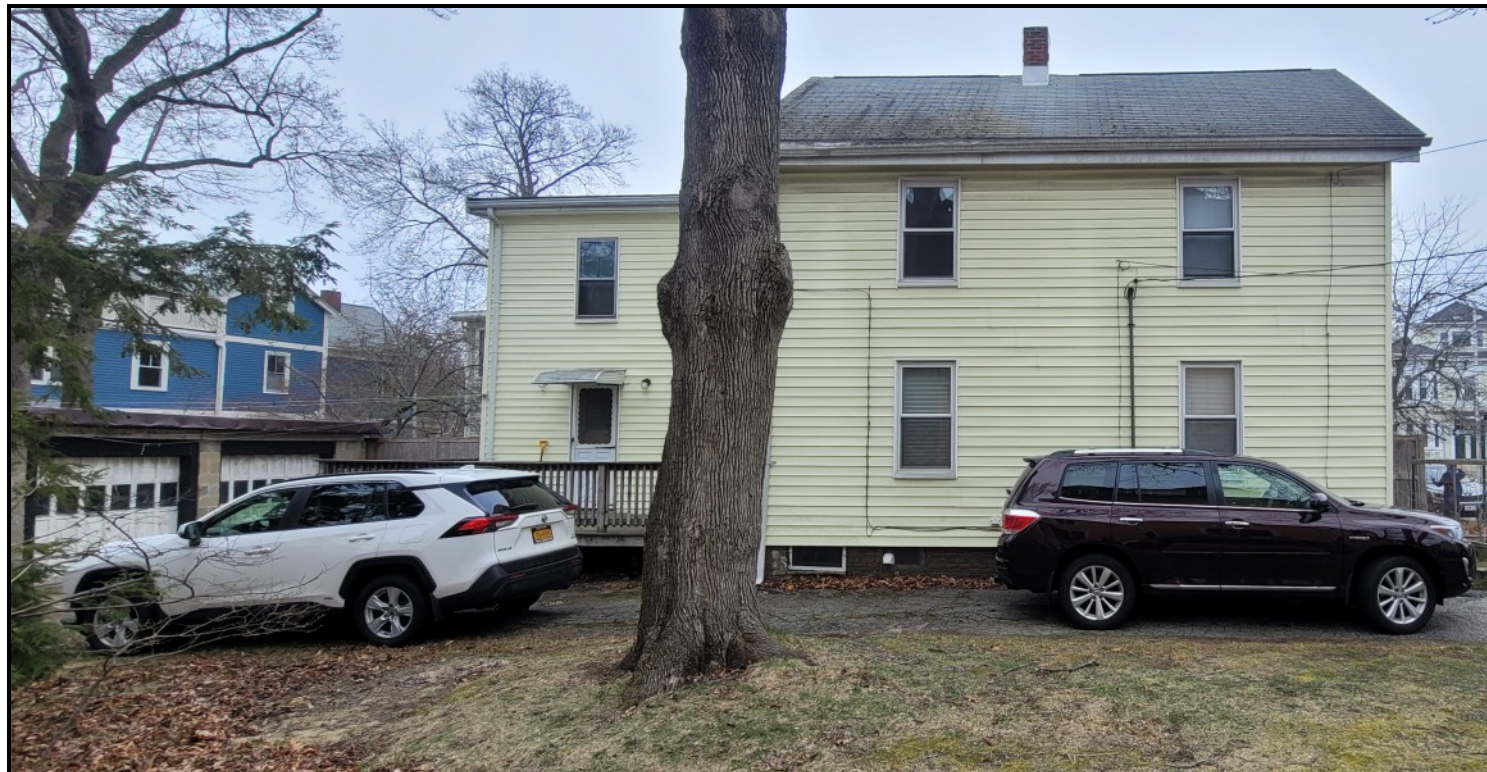
NW - Side Facade
