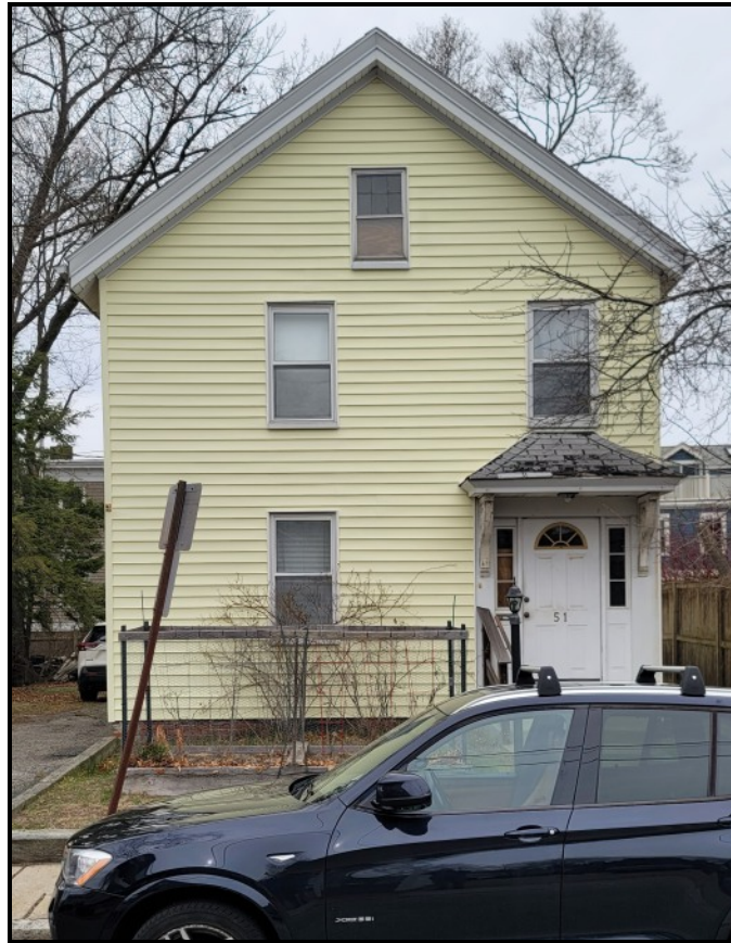
SW - Front Facade
