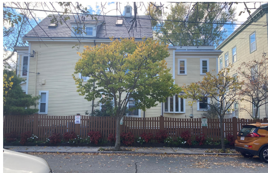
55 WENDELL ST - ELEVATION FROM GORHAM STREET
