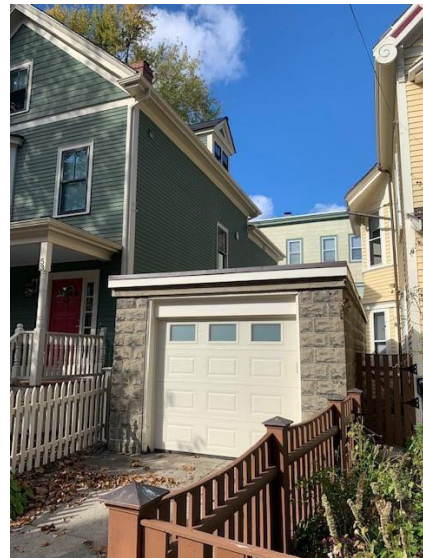
55 WENDELL ST - GARAGE
