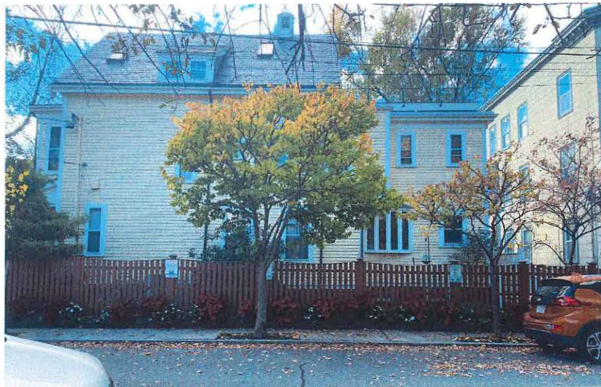
55 WENDELL ST - ELEVATION FROM GORHAM STREET
