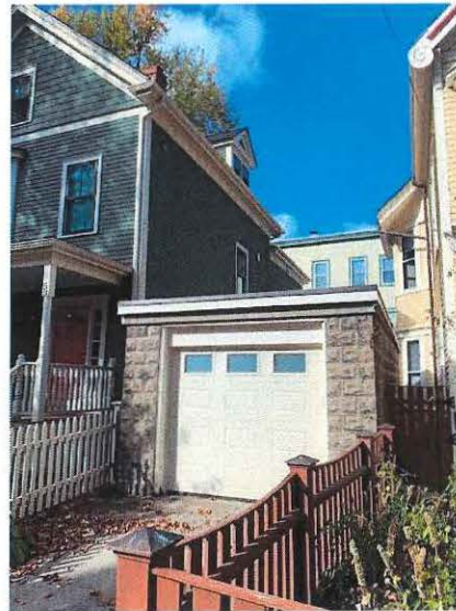
55 WENDELL ST - GARAGE
