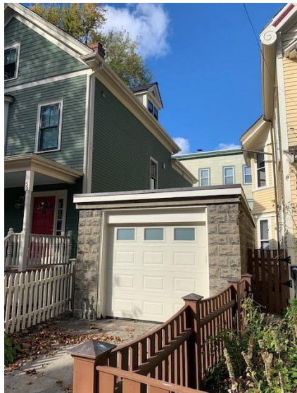
55 WENDELL ST - GARAGE
