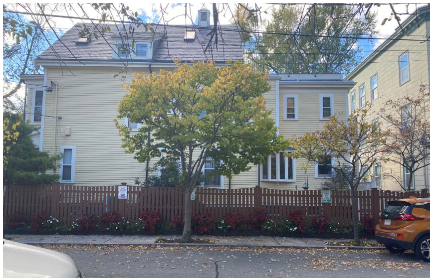
55 WENDELL ST - ELEVATION FROM GORHAM STREET
