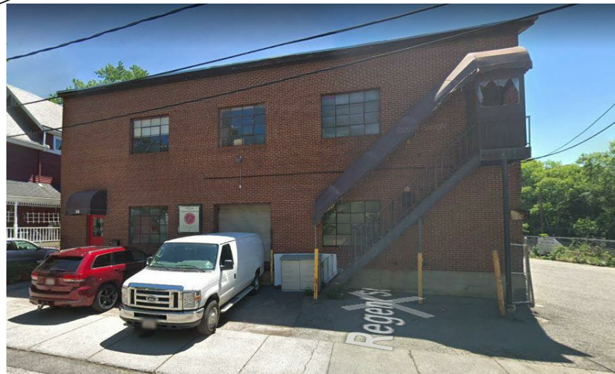
56 CREIGHTON, VIEW FROM CREIGHTON ST
