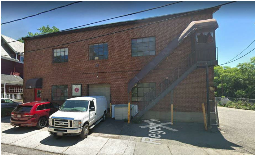
56 CREIGHTON, VIEW FROM CREIGHTON ST
