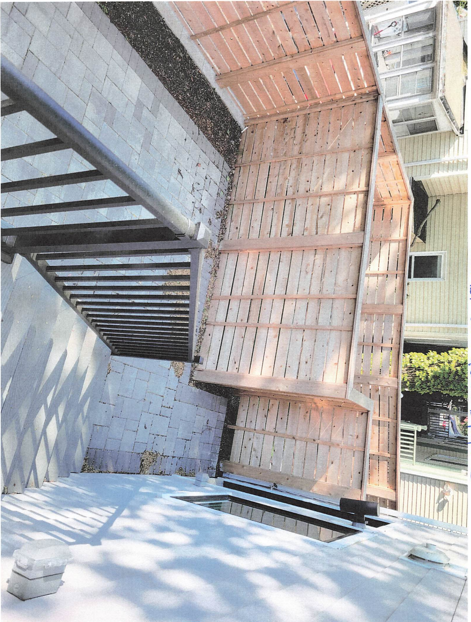
Roof frame where elevation is proper all
