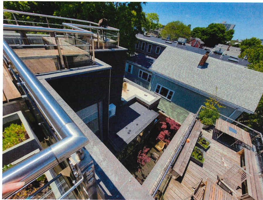
3 WEST SIDE, PHOTO FROM ROOF SCALE: NTS
