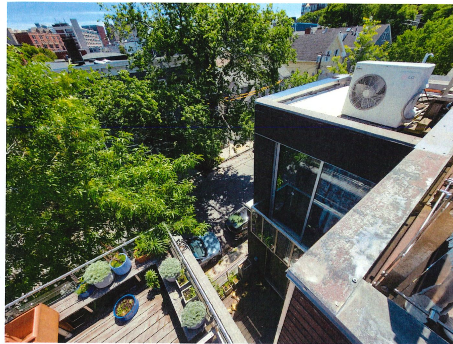
4 EAST SIDE, PHOTO FROM ROOF SCALE: NTS
