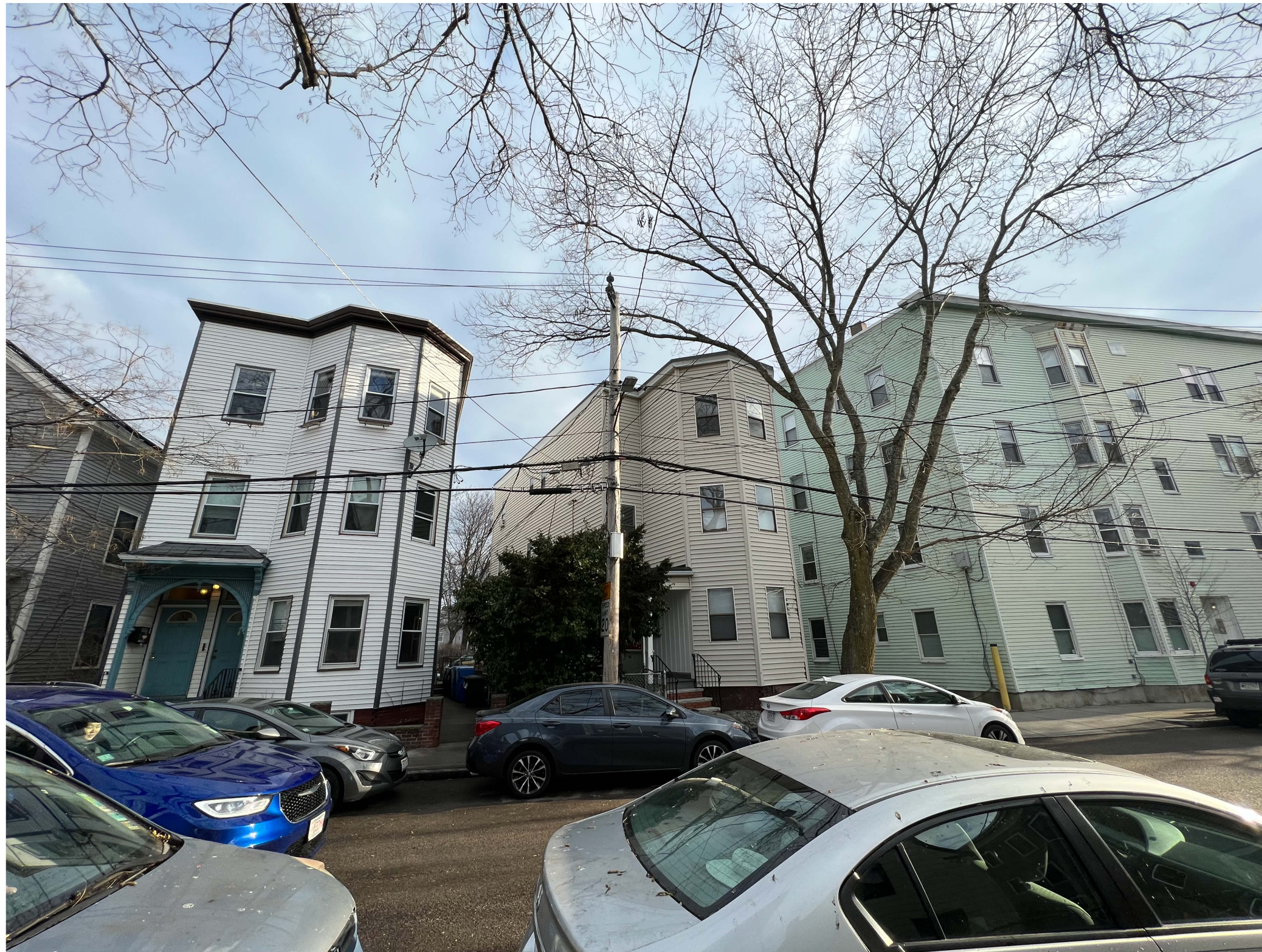
60 MARKET STREET VIEW DIRECTLY ACROSS THE STREET
