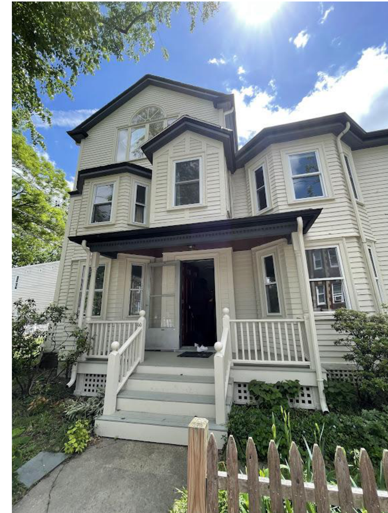
EXISTING VIEW FROM MARTIN STREET
