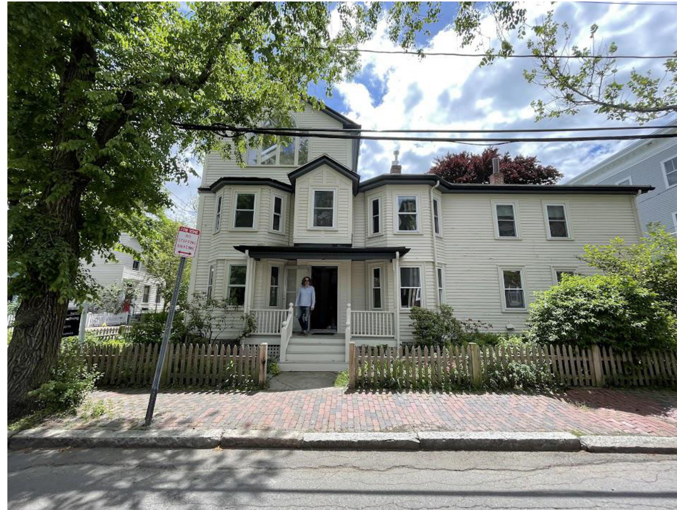
EXISTING VIEW FROM MARTIN STREET
