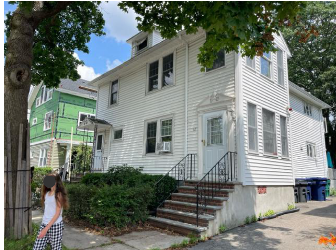
1 STREET VIEW FROM SOUTHWEST
