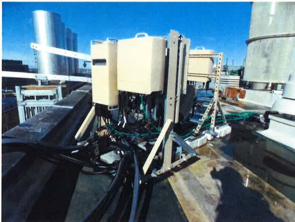
Photo 2: Sample photo illustrating the existing RRH ballast mount.
