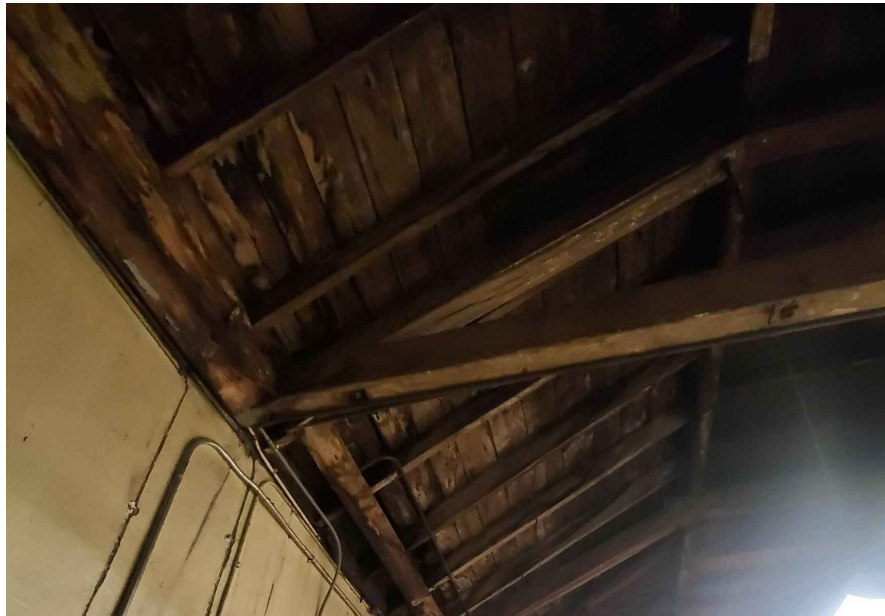
MIDDLE BUILDING EXISTING DETERIORATED ROOF STRUCTURE
