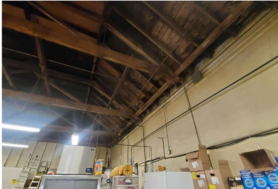
MIDDLE BUILDING EXISTING DETERIORATED ROOF STRUCTURE
