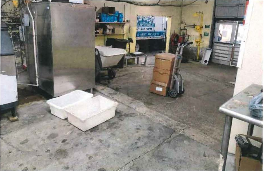
MIDDLE BUILDING EXISTING FLOOR SLABS
