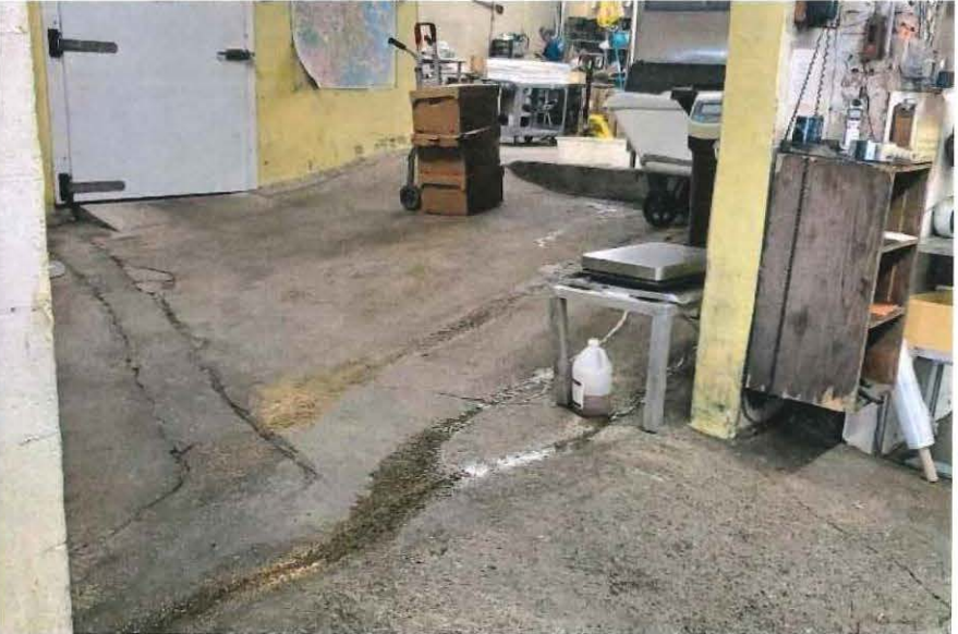
MIDDLE BUILDING EXISTING FLOOR SLABS
