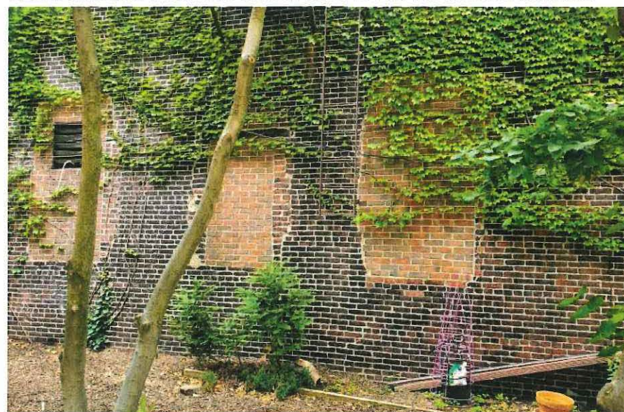
RIGHT - EXISTING WINDOW FILLINGS TO BE REOPENED
