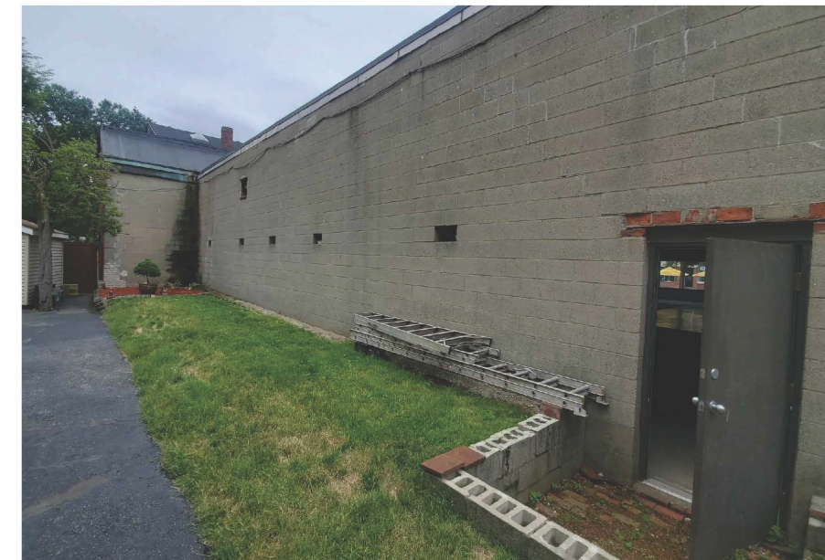
REAR ELEVATION EXISTING CONDITIONS- THIRD BUILDING
