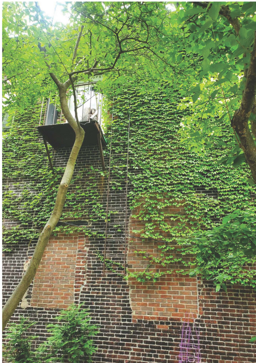
RIGHT - EXISTING FIRE ESCAPE AND EXISTING WINDOW FILLINGS
