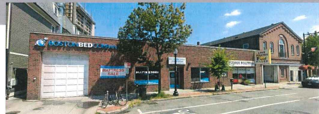
EXISTING VIEW EAST ON CAMBRIDGE STREET
