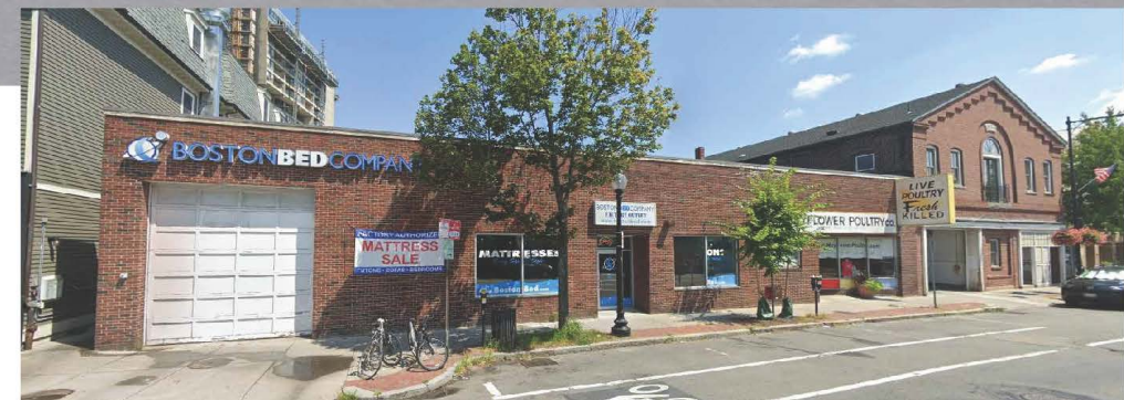
EXISTING VIEW EAST ON CAMBRIDGE STREET
