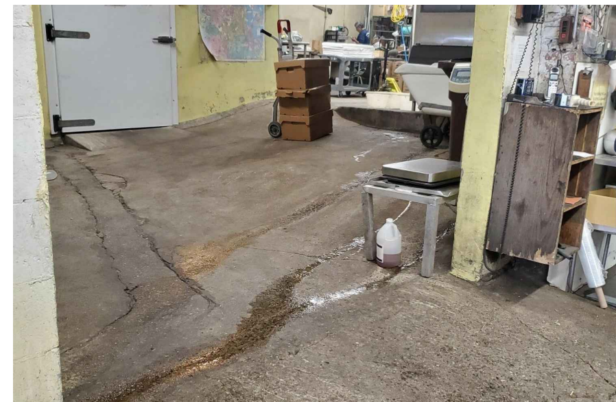
MIDDLE BUILDING EXISTING FLOOR SLABS
