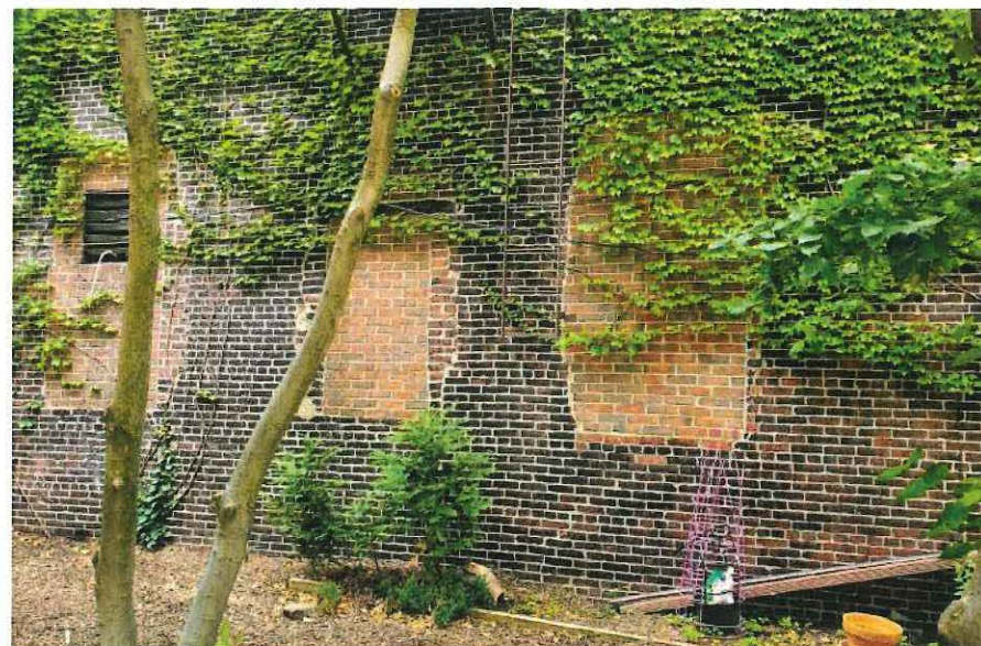
RIGHT - EXISTING WINDOW FILLINGS TO BE REOPENED
