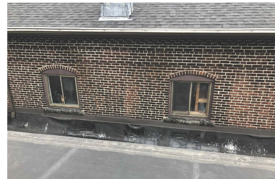
BARN LEFT SIDE - WINDOWS TO BE REPLACED
