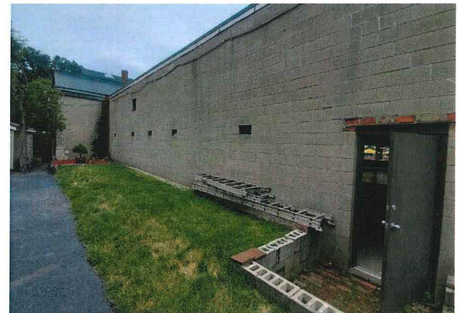
REAR ELEVATION EXISTING CONDITIONS- THIRD BUILDING
